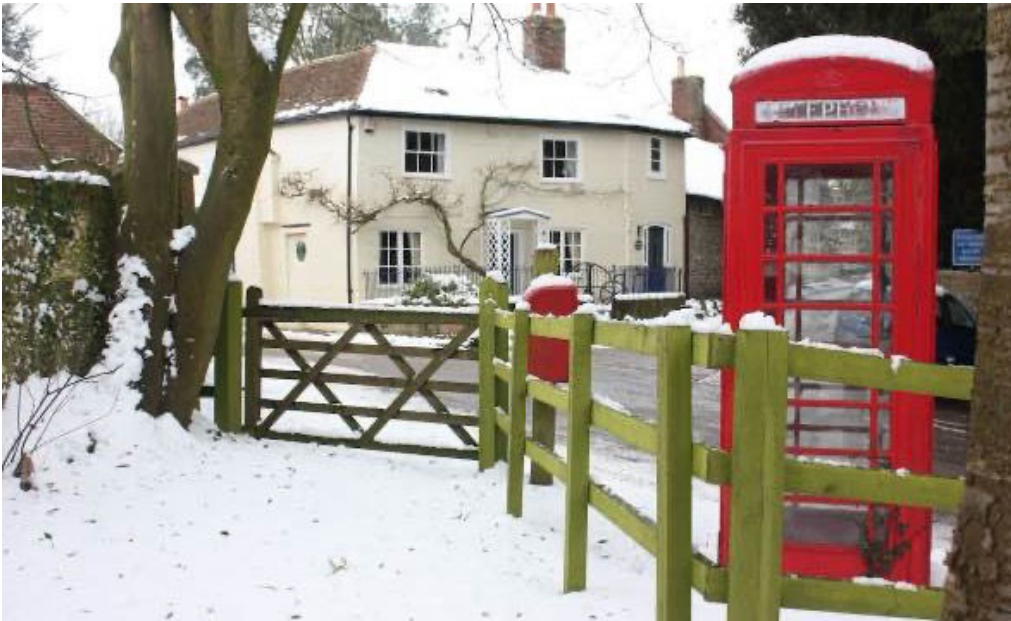
Photo 31. Pond House, Shoe Lane, with painted brickwork walls and former outbuilding in flint and red brick.
