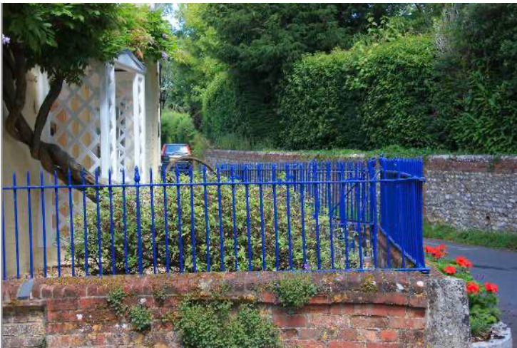
Photo 39. Simple painted metal railings at Pond House with brick and flint boundary wall beyond.
