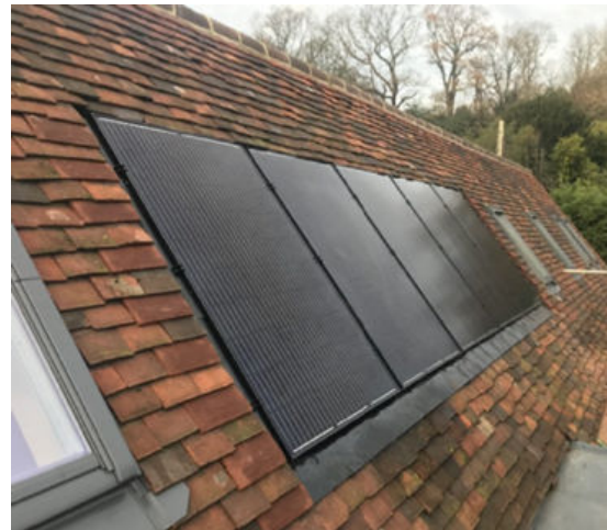
Photo 42. Solar Photovoltaic panels in a regular pattern and recessed into roof tiles.
