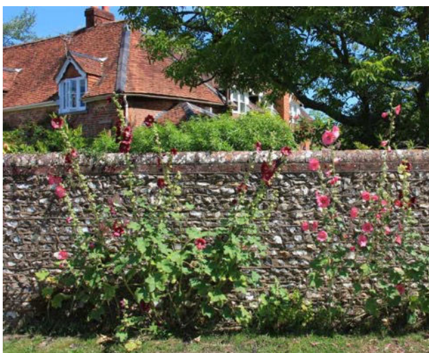
Photo 15. Flint and brick boundary wall in Shoe Lane.
