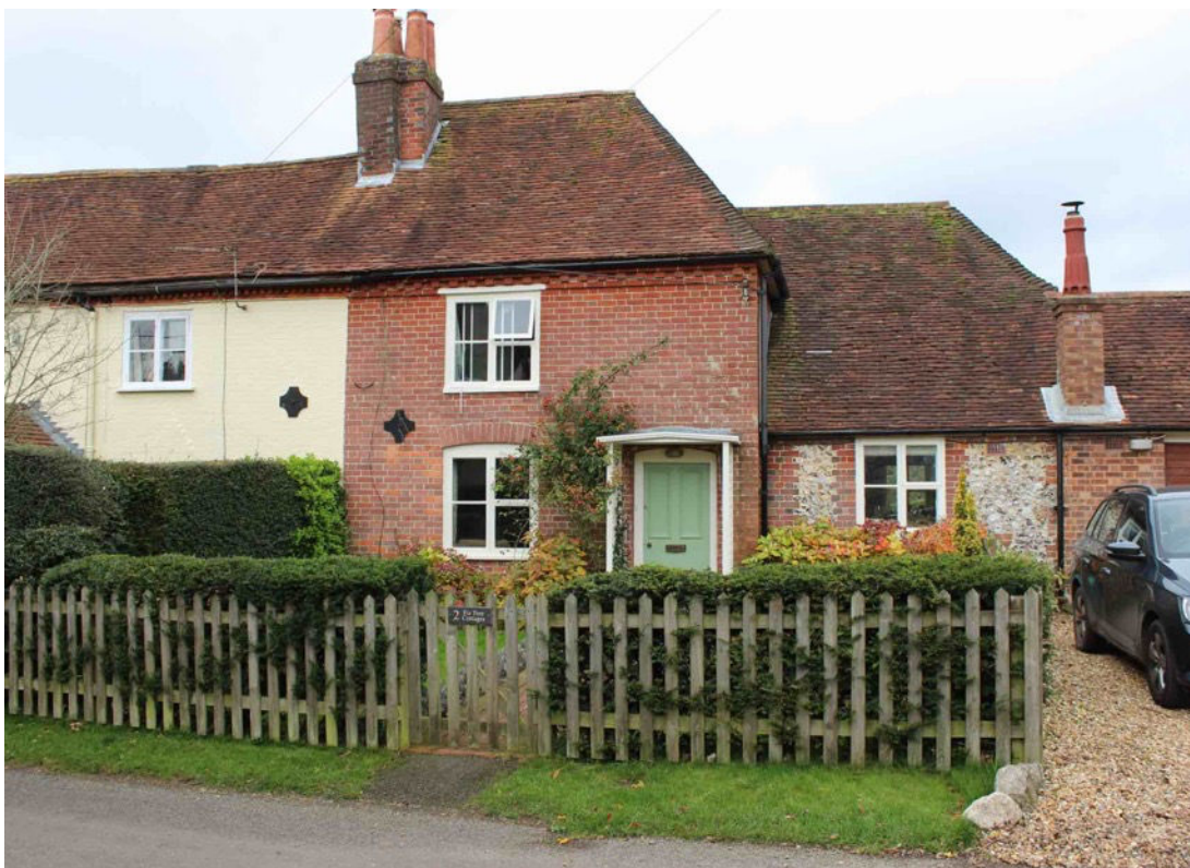
Photo 33. Cottages in Queen Street displaying walls of painted brick, plain red brick (unpainted) and flint and brick.
