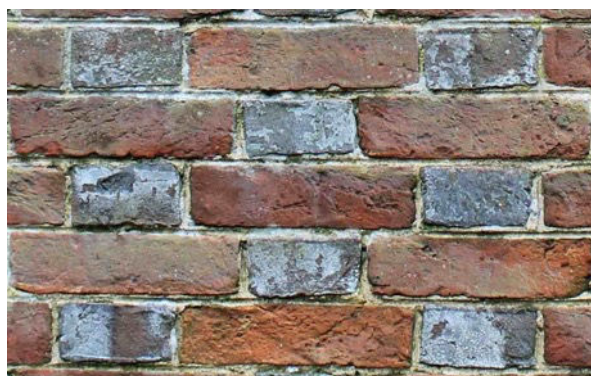
Photo 30. Brickwork in Flemish bond with red brick stretchers and grey/blue burnt headers seen on Upham Church and the Manor House and others.
