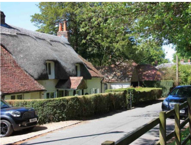
Photo 24. Little Croft on Church Street showing a variety of traditional building materials including thatch, clay plain roof and wall tiles, painted brick, and timber boarding.
