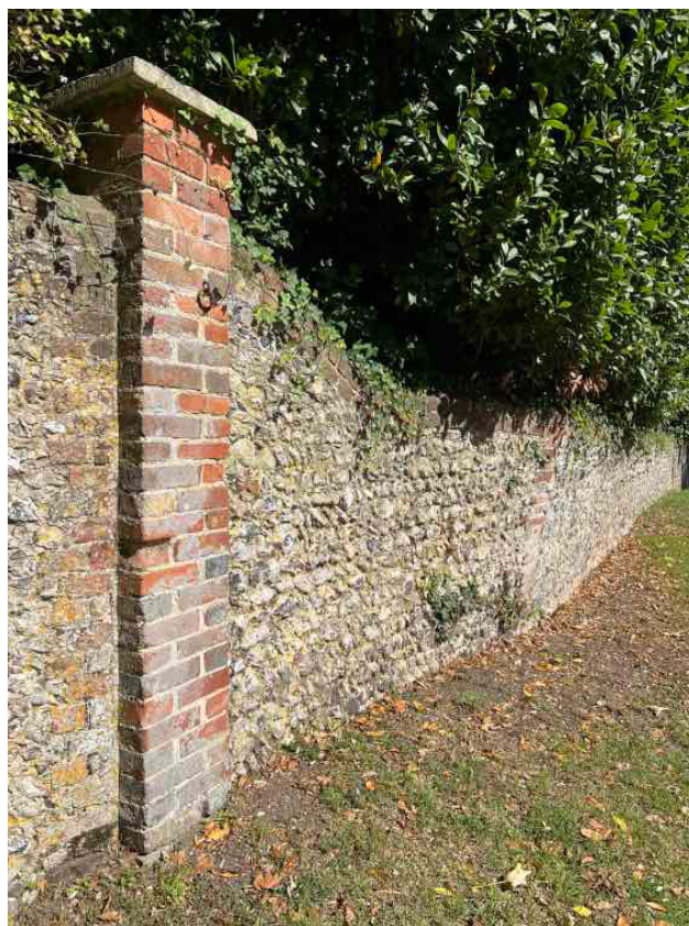
Photo 38. Typical brick and flint boundary wall at Holm House, Church Street.
