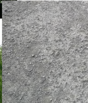
Previous old, degraded / uneven and broken sealed surface 2.5m wide
