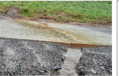
**Completed September 2024** New 2.5m wide path across former grazing fields , unbound gravel, limestone dust capped surface, new fencing / gates for land management.
