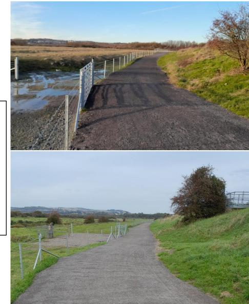
Completed September 2024 New 2.5m wide path across former grazing fields , unbound gravel, limestone dust capped surface, new fencing / gates for land management
