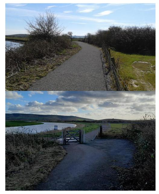
Completed September 2024 Vegetation clearance and surface cleared to re-establish 2.5m wide sealed surface.
