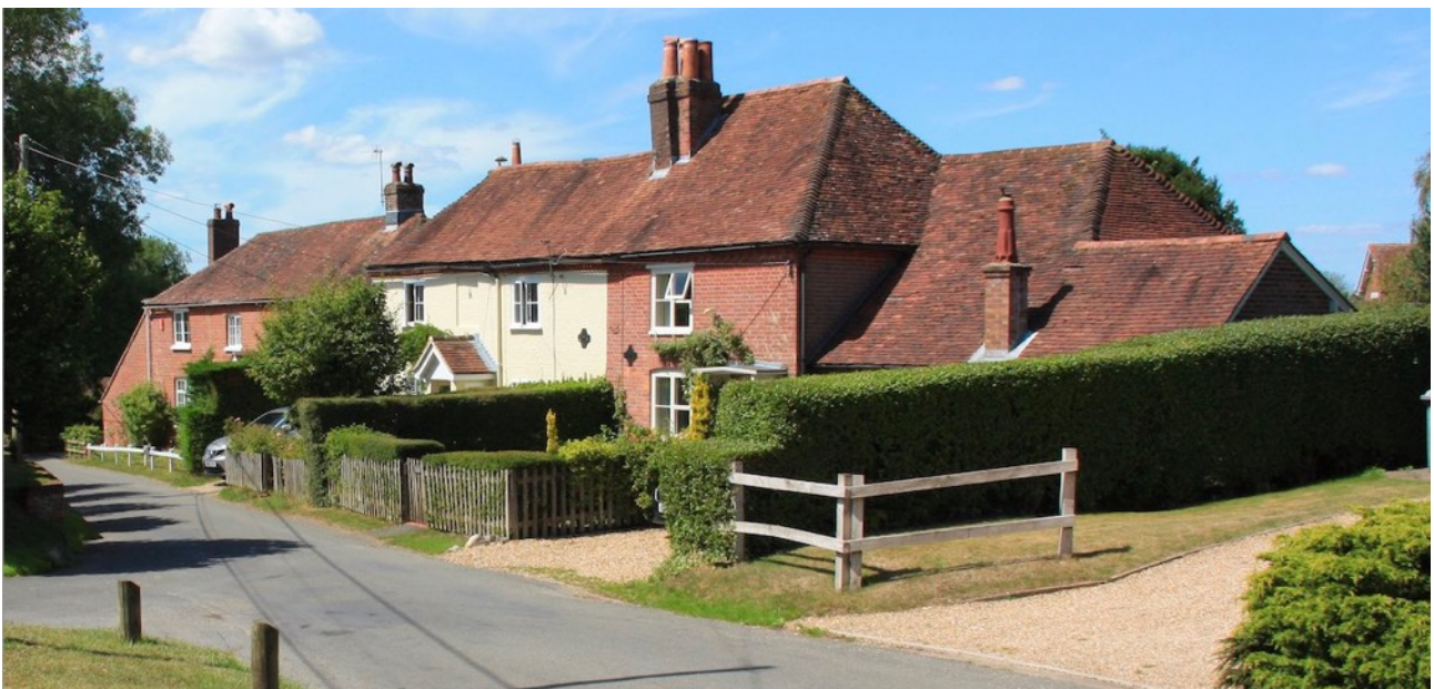
Photo 26. Houses in Queen Street with attractive silhouette and stepping roofline following the topography of the land.
