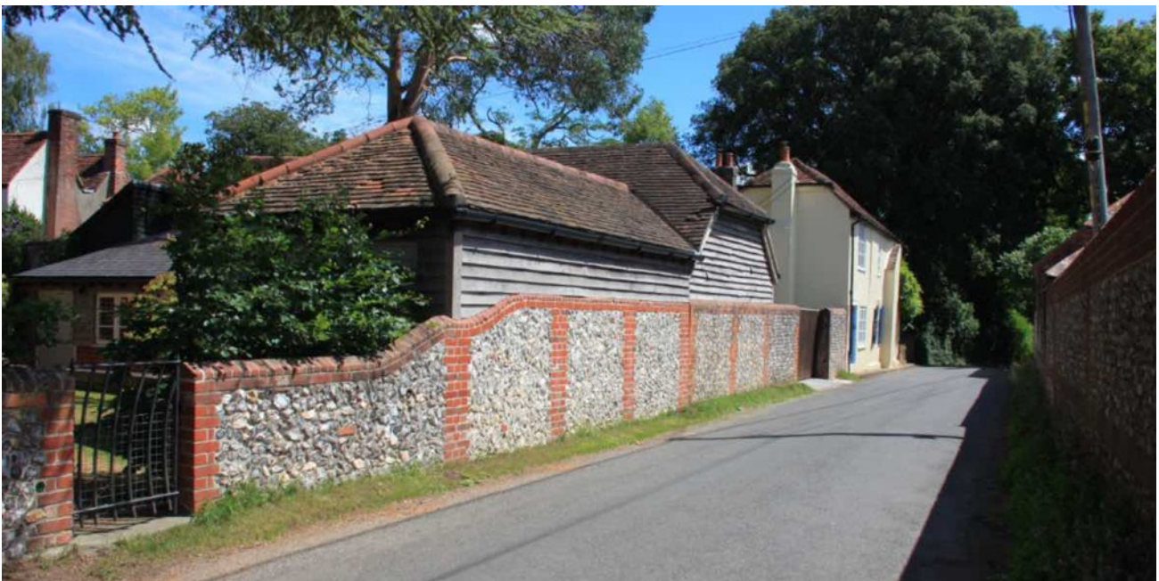
Photo 25. Outbuildings in Church Street subservient in scale and built using local materials that help to preserve the character of Church Street.
