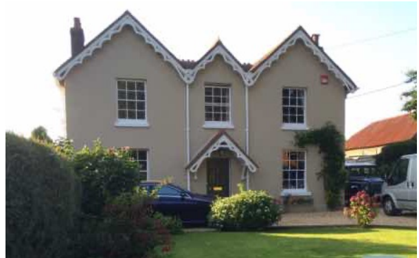
Photo 27. Gable ends facing the road are unusual in the village. The decorative barge boards are also not typical but add to the visual variety in the street.
