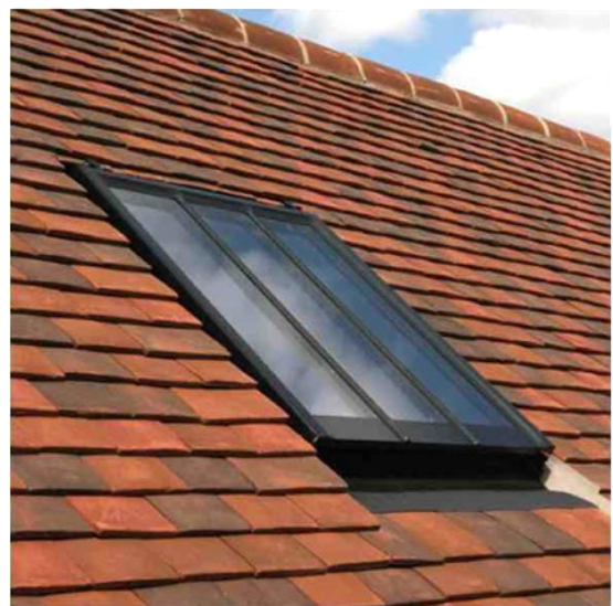
Photo 35. Conservation type skylight flush with roof surface
