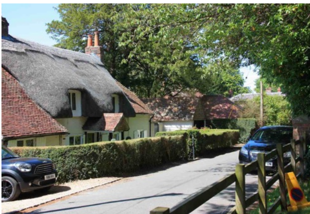
Photo 24. Little Croft on Church Street showing a variety of traditional building materials including thatch, clay plain roof and wall tiles, painted brick, and timber boarding.
