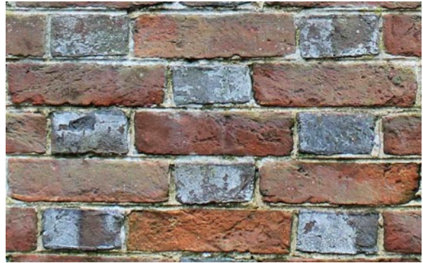
Photo 30. Brickwork in Flemish bond with red brick stretchers and grey/blue burnt headers seen on Upham Church and the Manor House and others.
