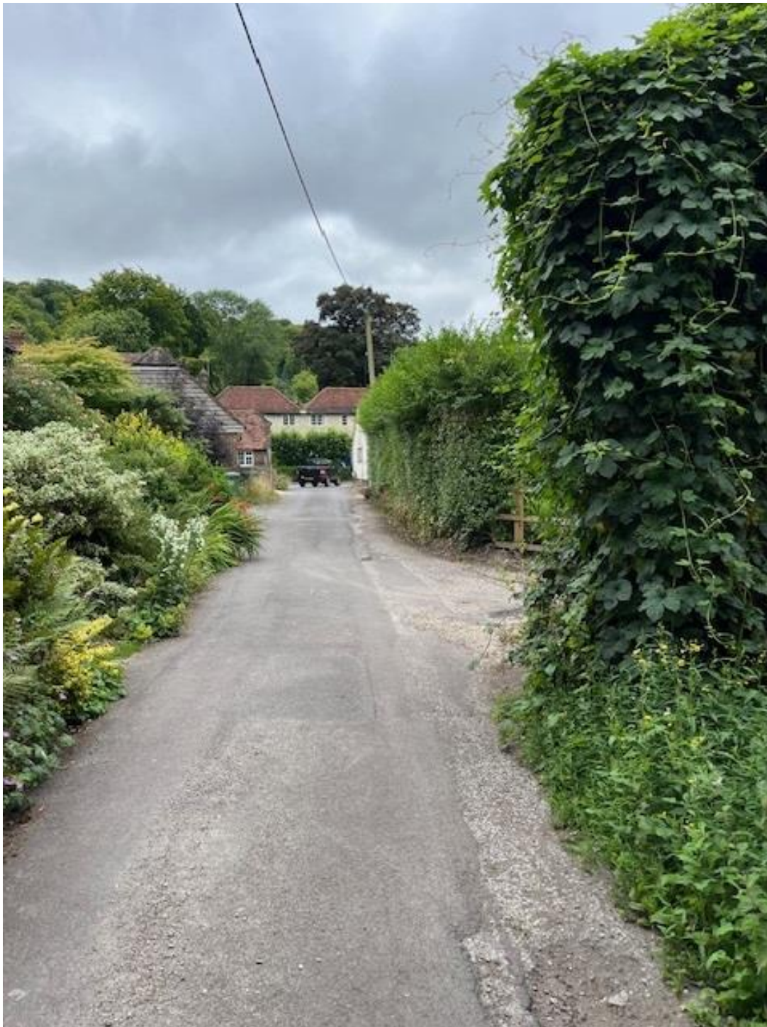
Photo.5 - View along Huckers Lane towards the High Street
