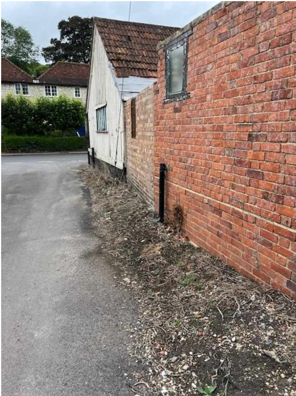
Photo.3 – Existing walls fronting Huckers Lane
