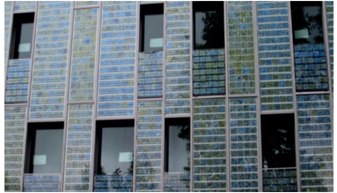
Rain screen cladding PV on an office building
