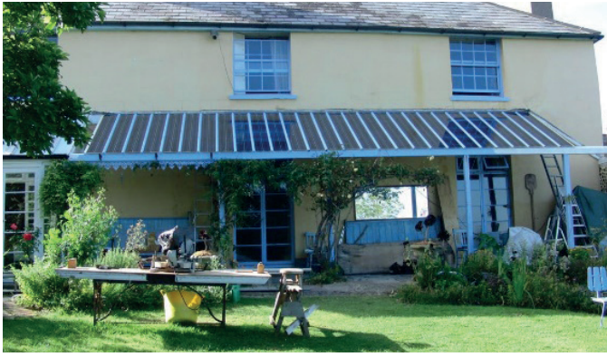
PV glazing in a discreet location
