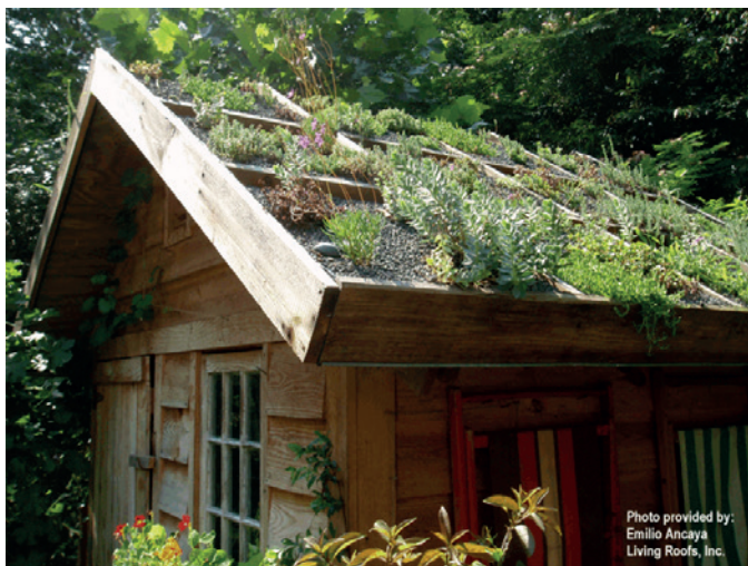
Green roofs on sheds and commercial buildings
