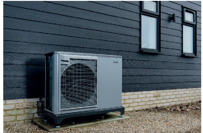
Air Source heat pump (Source: self-build.co.uk )
