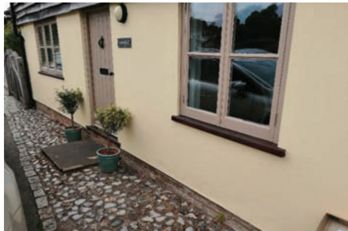
Figure 12.23: House in Hambleton showing how render is protected from ground splash back with brick detail.
