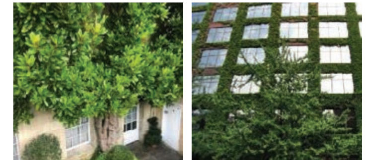
Figure 9.31 and 9.32: Extensive green walls of magnolia grandiflora and ivy on an office building in Edinburgh.
