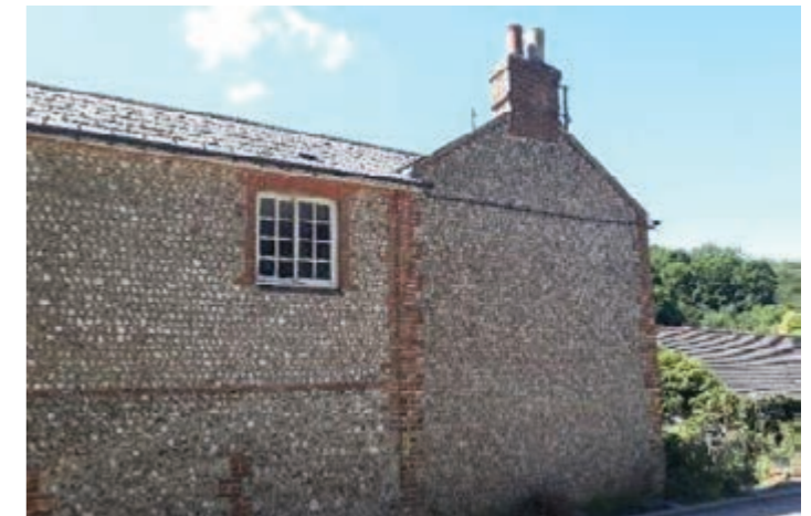
Figure 12.13: Flint building in Stanmer Park.
