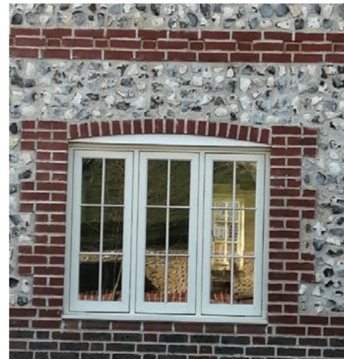
Figure 12.28: Locally characteristic brick window detailing in new East Dean development.
