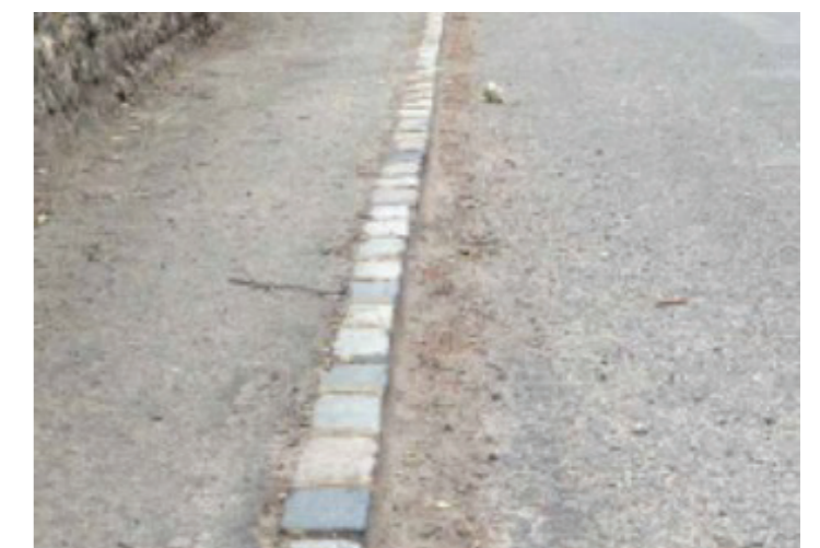
Figure 12.50: Setts are used to define the footway in Selborne.
