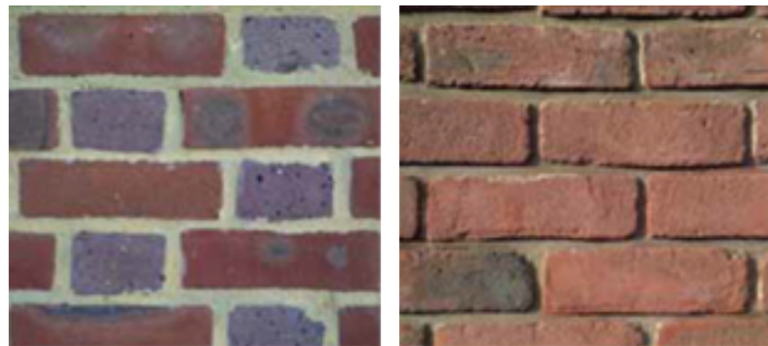
Figure 12.5: Mortar coursing has a profound effect on the appearance of brickwork.
