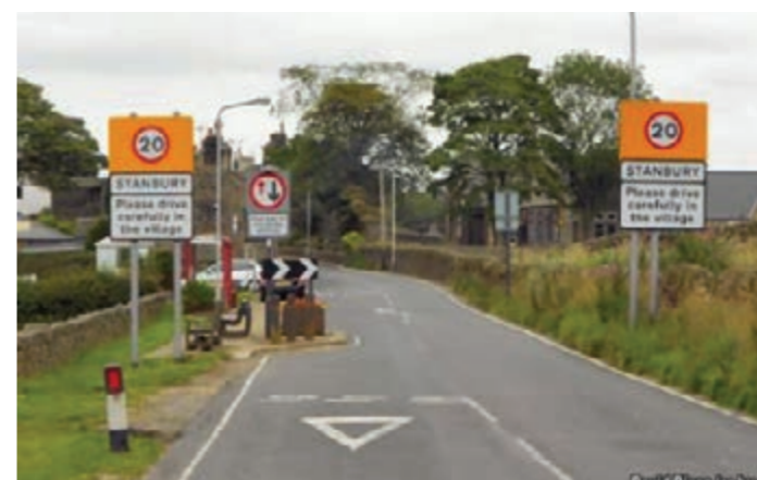
Figure 7.5: A poor example of an over-designed village gateway with an inappropriately cluttered result.
