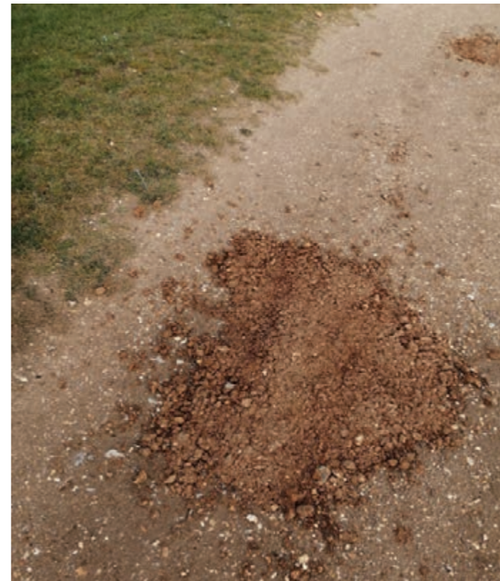
Figure 12.56: Hoggin footpath being repaired with fresh material and prior to compaction, Hampshire.
