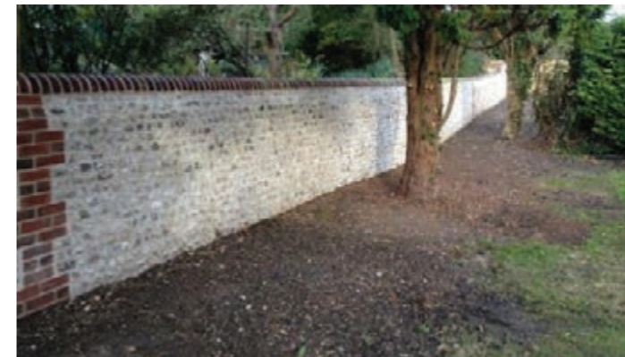
Figure 12.9: A well built, new flint wall with masonry piers and coping.
