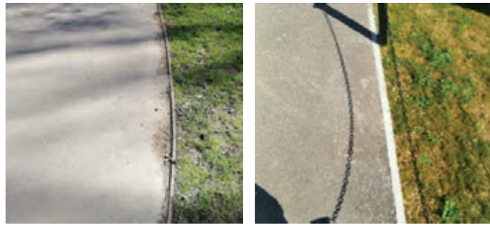
Figure 12.51: Timber edge detailing (Midhurst, left) has a more low-key visual impact than concrete pin kerbs (Cheriton, right). Timber can be more appropriate in rural contexts or where a more 'natural' approach is called for.
