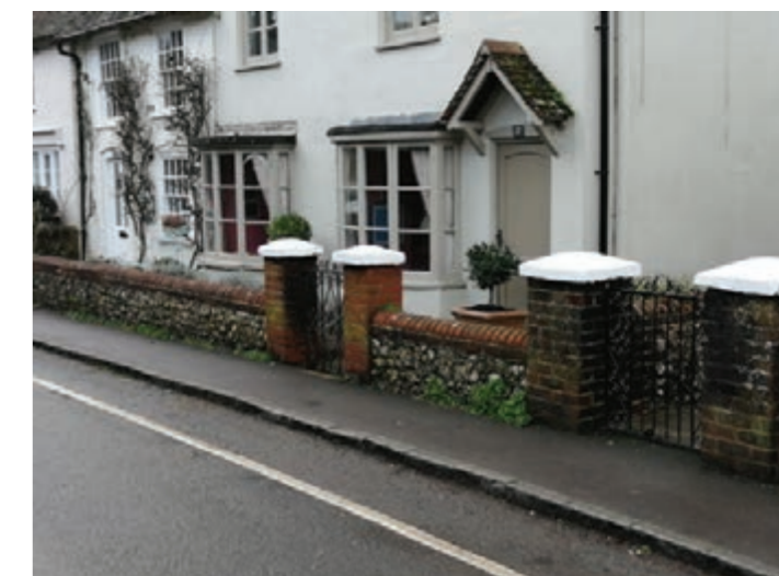
Figure 11.4: Front garden walls in Buriton in local stone (flint) and brick with pedestrian gates.
