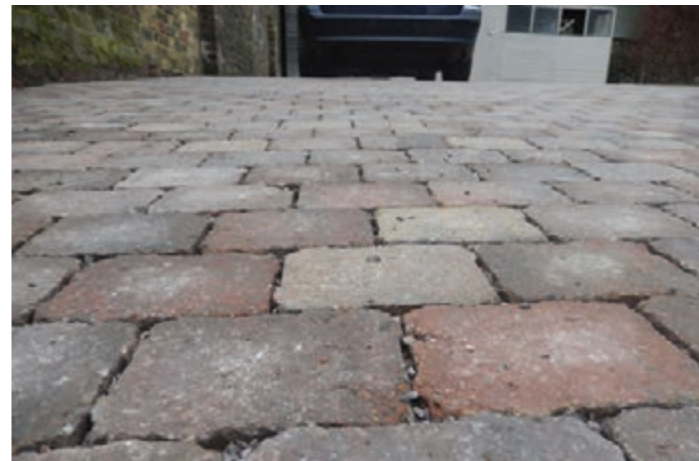
Figure 12.48: Permeable block paving on a private drive is designed with nibs to keep gaps between blocks open to allow water infiltration.
