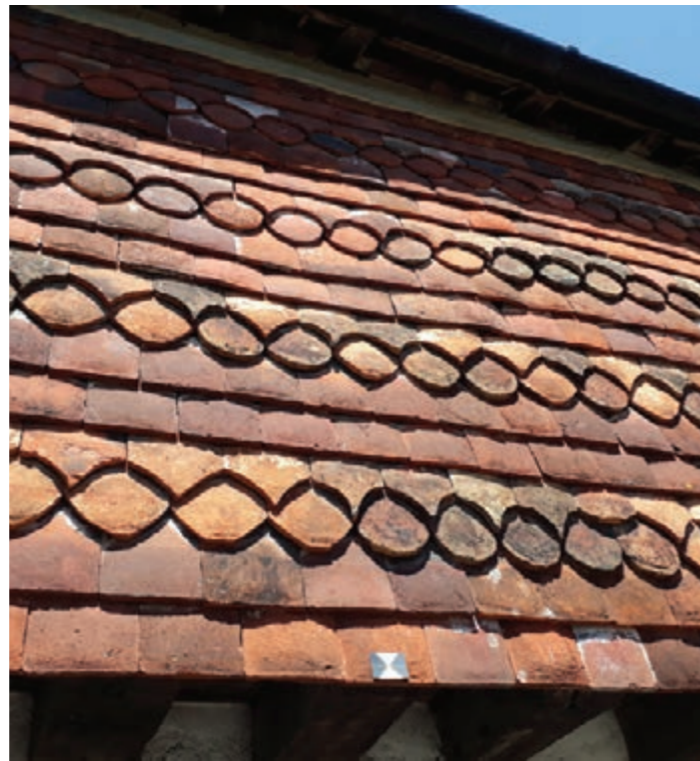
Figure 12.19: Clay hanging tiles in Alfriston.
