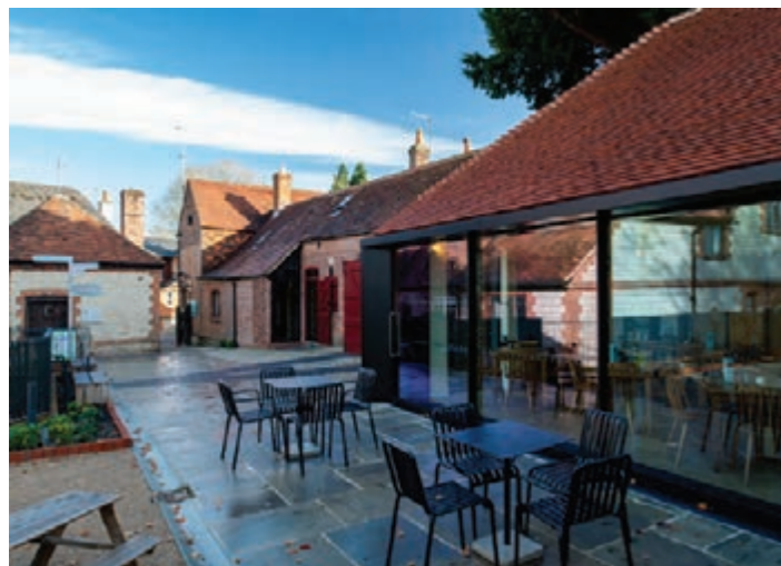
Figure 13.7: Gilbert White Museum successfully marries refurbished listed buildings with a contemporary style extension.
