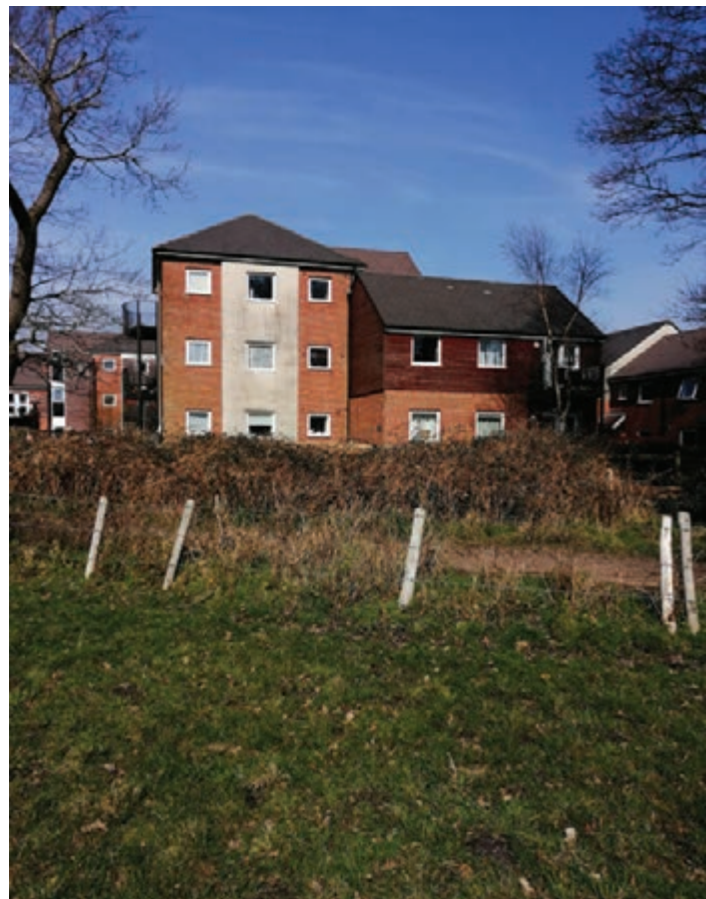
Figure 1.17: Inappropriate building height, form and materials on countryside edge.
