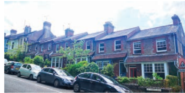
Figure d: Good example of buildings following contours in Lewes.
