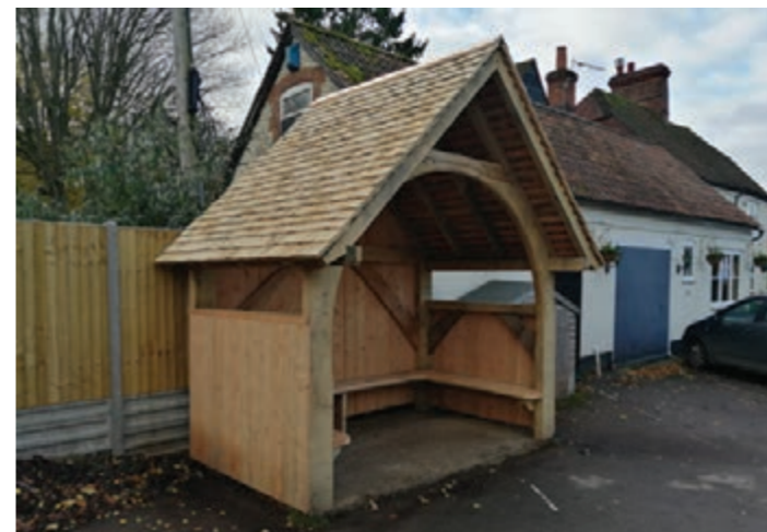
Figure 8.26: An attractive bus shelter in Selborne with a traditional timber construction and timber shingle roof.
