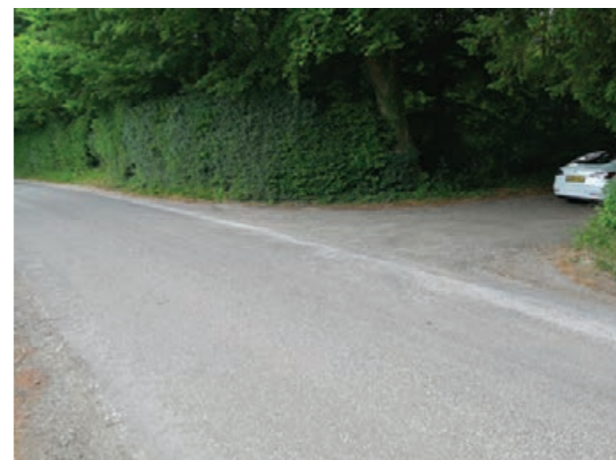
Figure 7.4: Appropriately low-key access to several properties on same road as Figure 7.3 with modest access width, short break in hedge line, no kerbs and stone surfacing.
