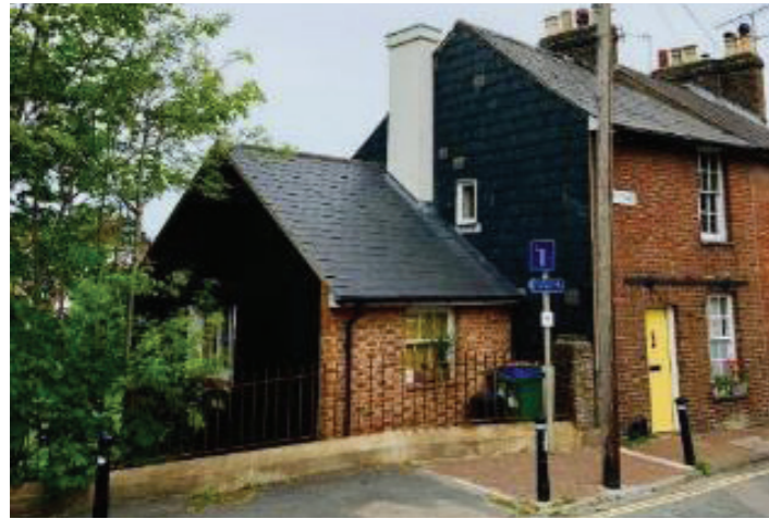
Figure 12.16: Vertically hung slate tiles in Lewes.
