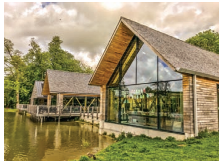
Figure 12.26: locally sourced cedar roof shingles are used on buildings at The Weald and Downland Museum.
