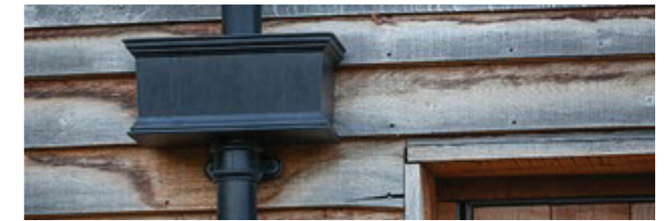
Figure 12.29: Aluminium rainwater goods (Guttercrest).
