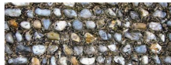
Figure 12.12: Galletted flint (flint shards incorporated into the mortar).
