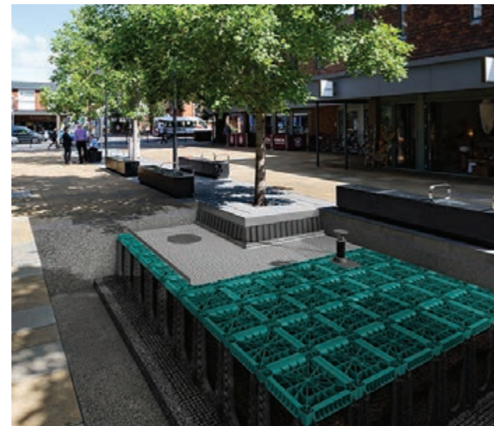
Figure 9.16: An example of a cellular system under a street (GreenBlue Urban).
