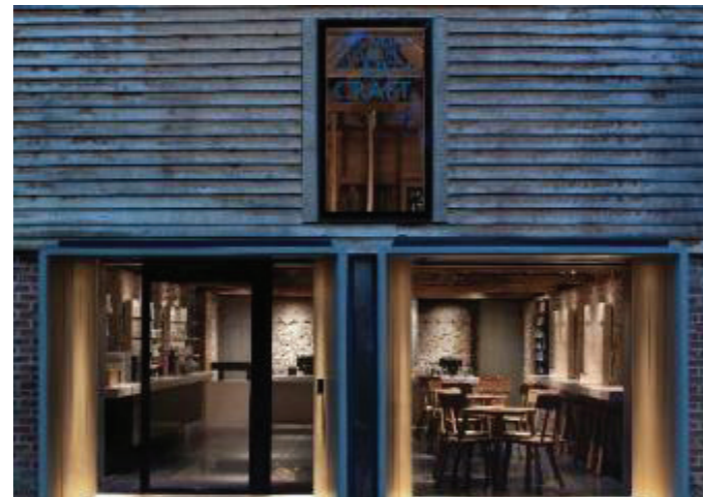
Figure 12.25: Horizontal timber cladding used in a contemporary building (Ditchling Museum of Art and Craft).
