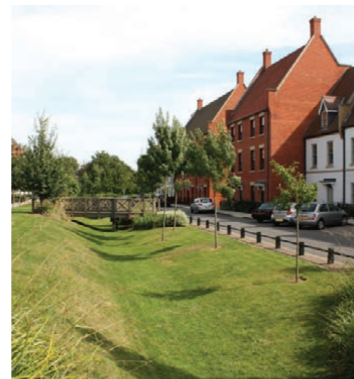
Figure 9.19: Swale in new housing development (Ciria SuDS Manual).
