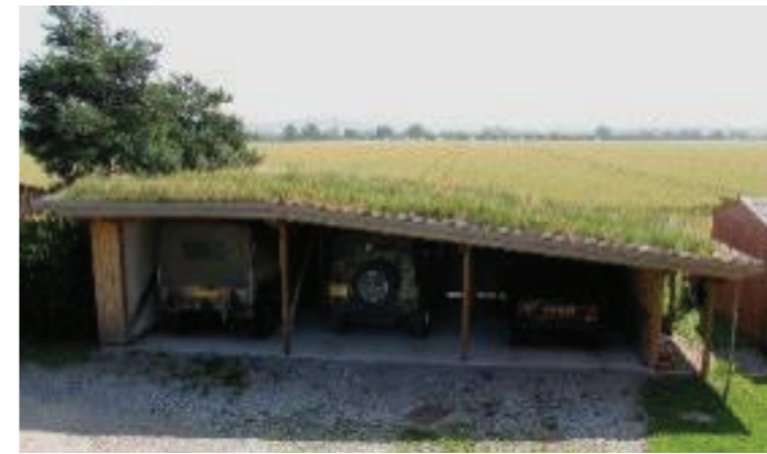
Figure 9.29: A green roof car port (DIY green roofs).
