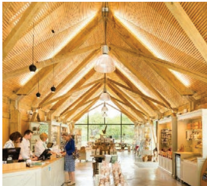
Figure 12.24: Locally sourced oak timber frame.
