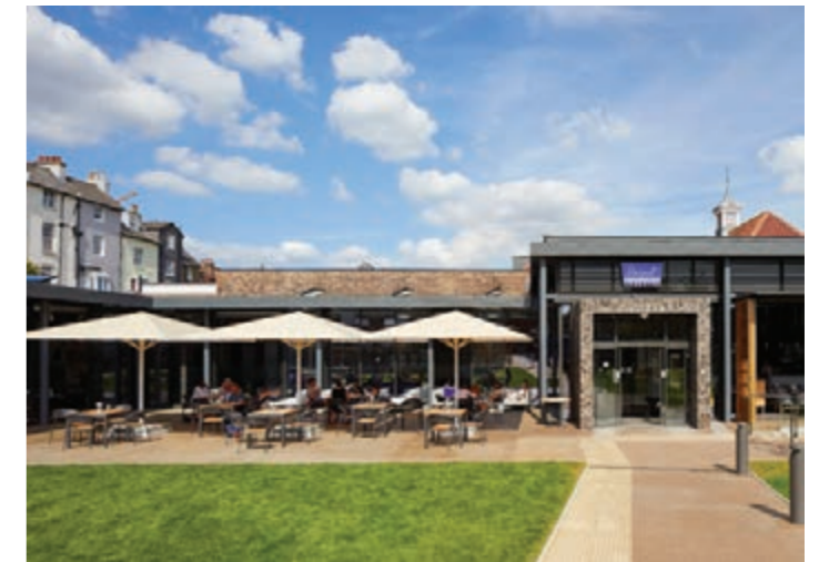
Figure 13.30: Main entrance at the Depot, Lewes is emphasised by flint door frame and external works.
