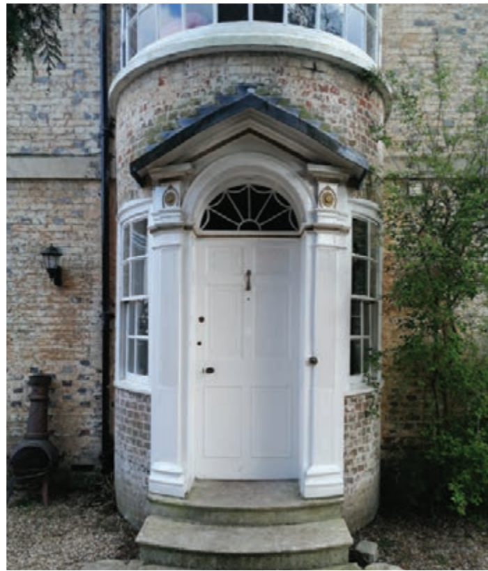
Figure 13.25: A good example of a doorcase on a house in West Meon, with the gate reinforcing the entrance experience.
