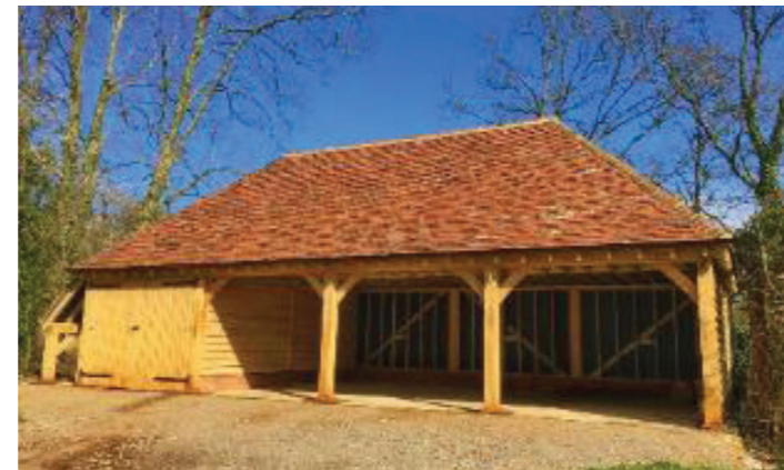
Figure 8.8: A car barn using local traditional building style and materials.
