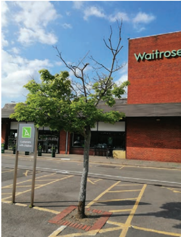
Figure 9.15: Supermarket car park: Trees failing after a few years due to inadequate root soil volume and compaction.
