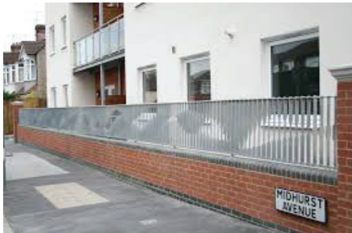
Figure 12.36: Newly built brick and simple galvanised railing boundary structure in a contemporary style development.
