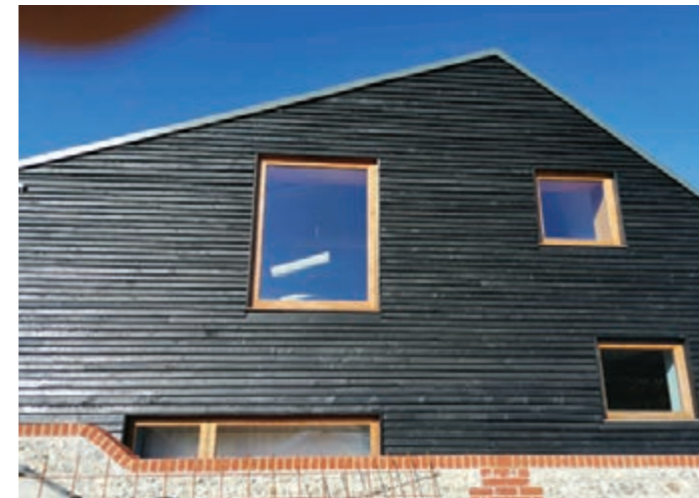
Figure 12.27: A contemporary designed new home in rural West Sussex uses dark stained horizontal timber cladding which references a locally common agricultural building material.
