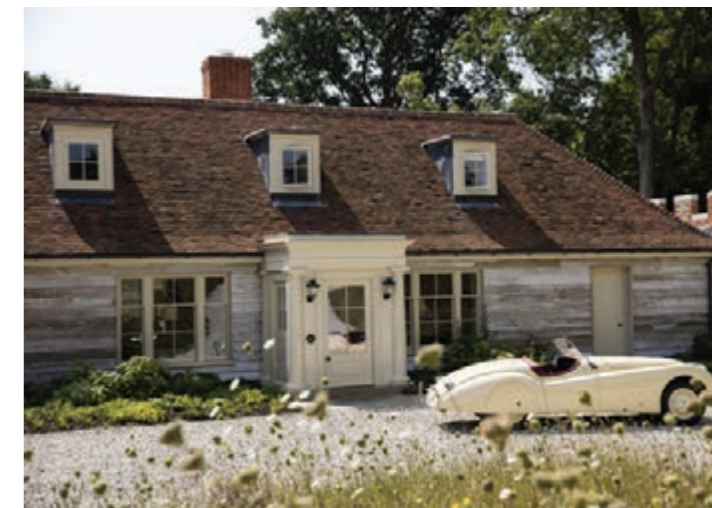
Figure 13.3: The dormers in this new development at the Goodwood Estate demonstrate dormers in perfect proportion to the rest of the roof and the building.
