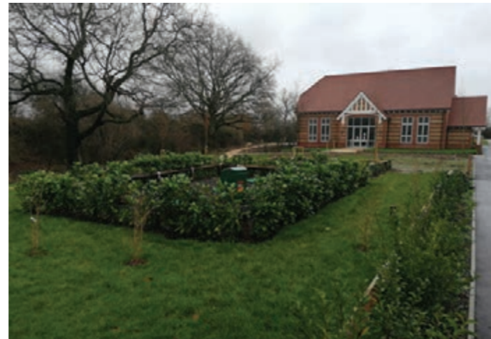
Figure 8.24: Gas plant poorly located in a prominent position on the approach to residential development and using inappropriate suburban character screen planting, Stroud.
