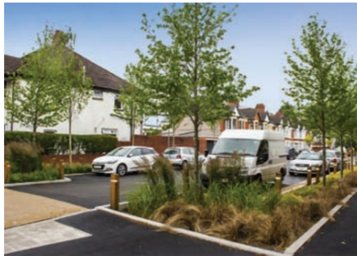
Figure 14.12: Rain garden and street trees help adapt streets to predicted climate change.
