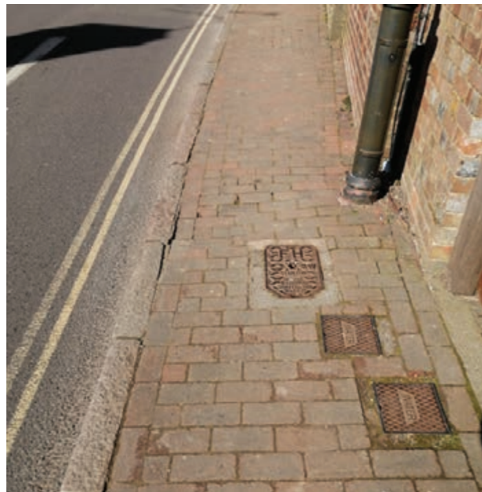
Figure 12.46: Concrete block pavers (here 'Tegula' in Petworth) are widely used in more urban contexts. This can lead to an 'anywhere' character whereas local stone or clay pavers are preferable as they reinforce local character.
