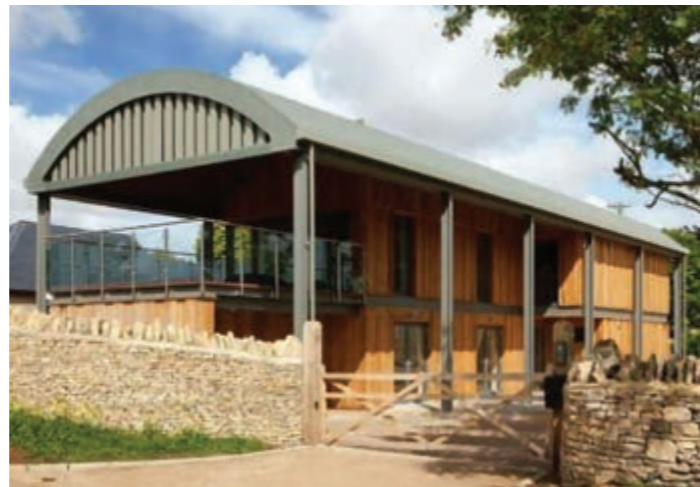
Figure 5.5: Successful conversion of steel framed open cattle shed in Devon.
