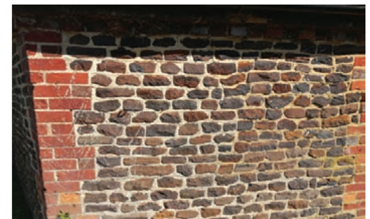
Figure 12.15: Ironstone house, Greatham.
