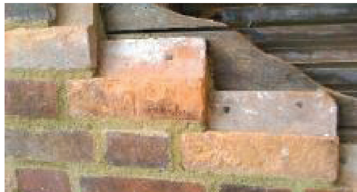
Figure 12.17: Mathematical tiles being attached.
