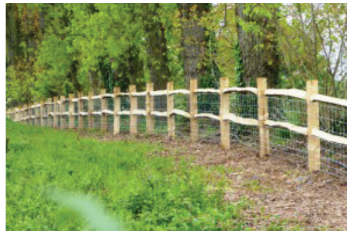
Figure 12.38: Chestnut cleft post and rail fencing with wire mesh animal proof fencing attached.
