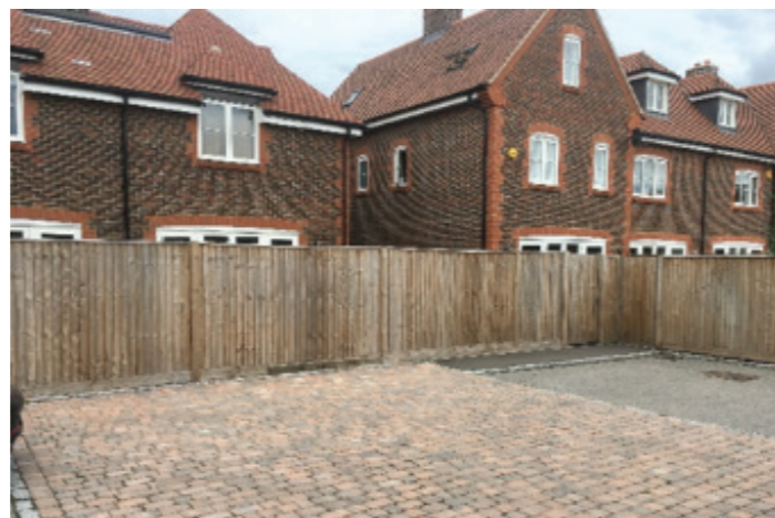
Figure 11.1: Close board fences between very small rear private gardens and car parking, Midhurst, provide only minimal acoustic insulation.
