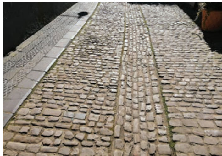
Figure 12.44: A simple design of Stone setts with central channel and blue, clay paver side detail make a beautiful place in a Petworth pedestrian street. The uneven texture may cause problems for some users.
