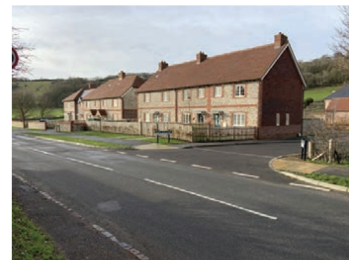
Figure 7.7: An inappropriately over-engineered new access at East Dean.
