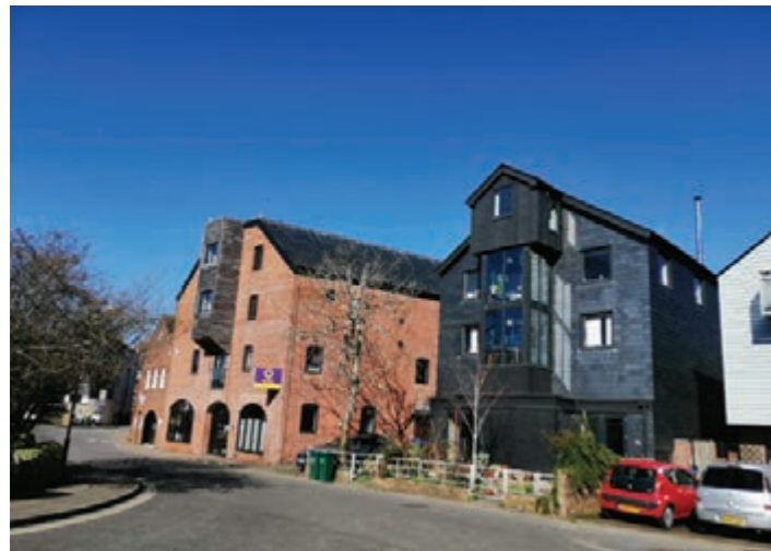
Figure 13.1: Existing traditional river warehouse buildings converted sympathetically for residential use. The new buildings in Figure.13.2, on the same river, reflect a similar scale and form.
