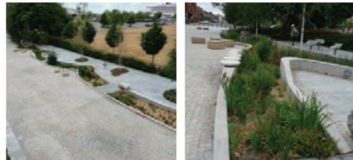
Figure 9.25: A rain garden in Southampton city centre.
