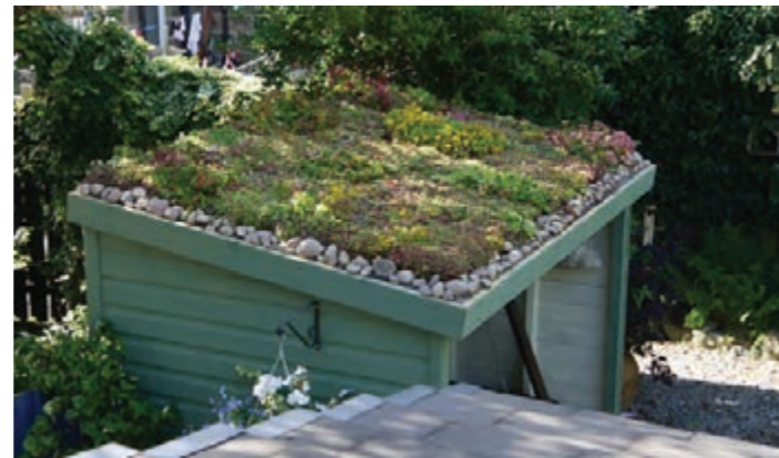
Figure 9.28: Sedum green roof on a garden shed.
