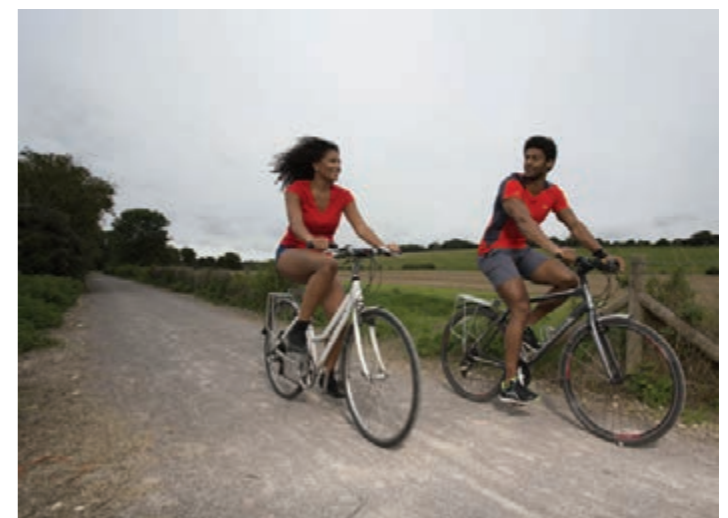
Figure 12.42: Centurion Way between Chichester and West Dean is a good example of a rural cycle (and pedestrian) route with a very simple construction using local materials. (A self-binding limestone dust over a 'Type 1' graded stone sub-base with no edge details or kerbs).
