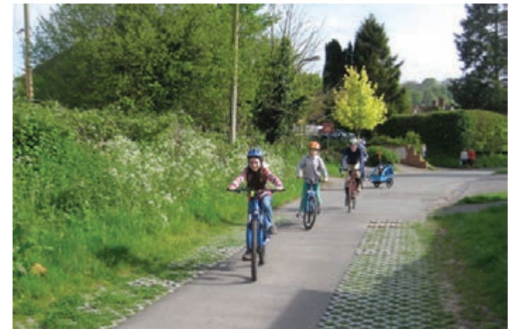
Figure 12.40: Reinforced grass paving used in Buriton to visually narrow the road while allowing for occasional wide vehicles.
