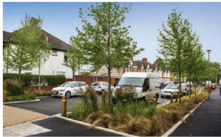
Figure 8.2: The visual impact of cars in traditional on street parallel car parking in a suburban street is successfully mitigated with rain gardens and street trees.
