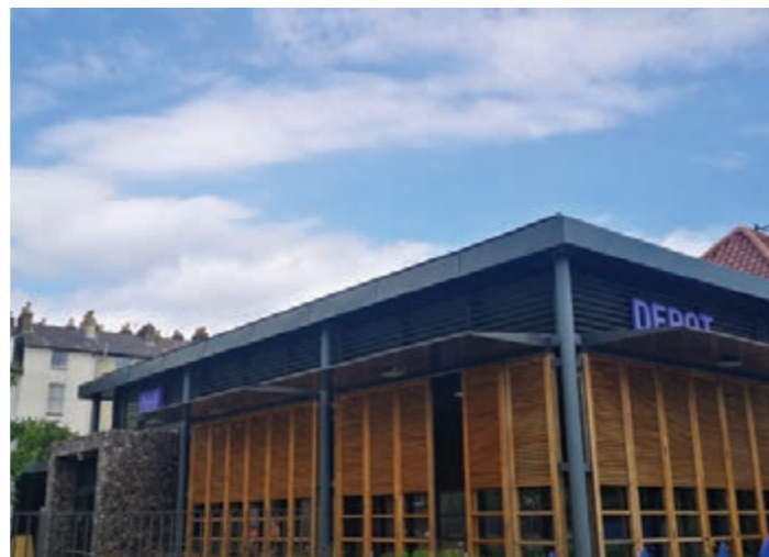
Figure 15.2: The Depot in Lewes uses external blinds to mitigate the effects of large windows at night.
