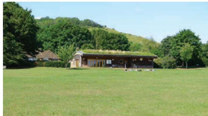
Figure 9.27: Green roof on sports pavilion, Kingston.
