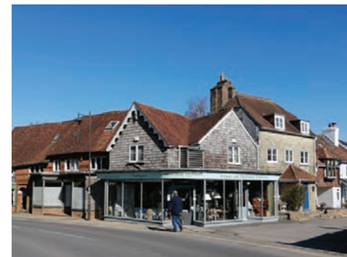
Figure 12.3: An example in Petworth of how a variety of traditional elevation materials (hanging clay tiles, timber shingles and local stone) on different buildings is brought together under a consistent use of red clay roof tiles.
