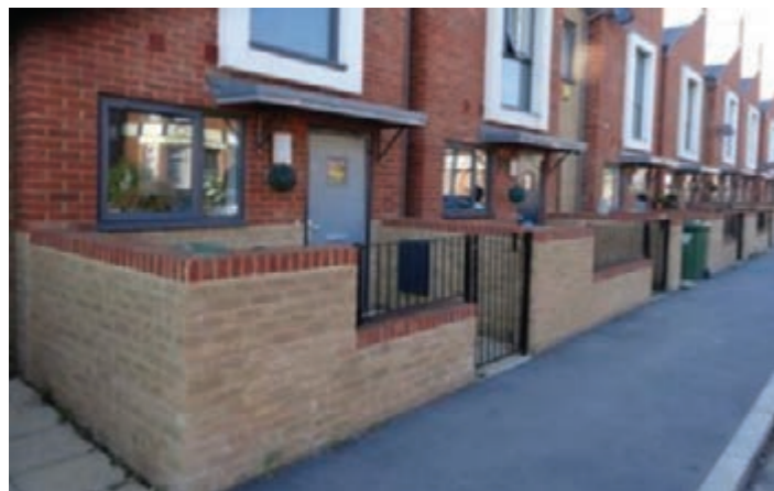
Figure 11.7: Front garden walls screening bins in terraced houses, Hampshire.
