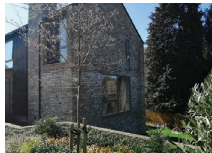
Figure 13.21: A good example of well-proportioned and crisply detailed windows in a contemporary design building, Selborne.
