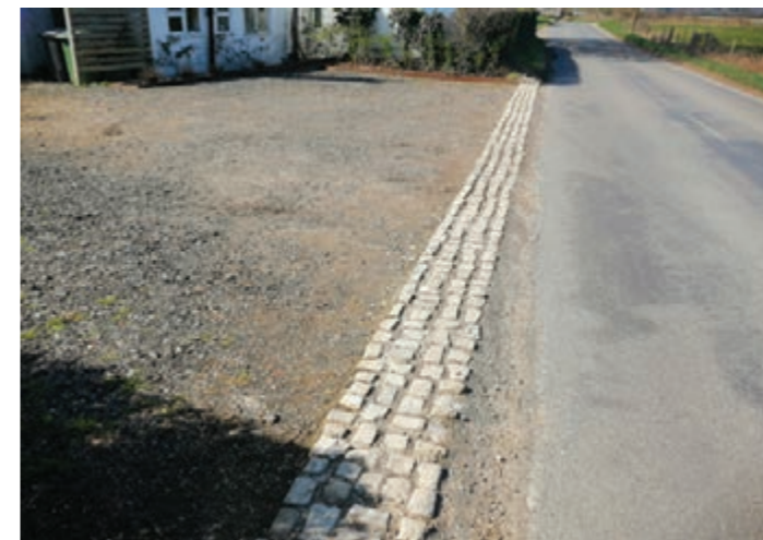
Figure 12.39: Courses of granite setts create an appropriate and robust edge between a rural road and a private, stone-surfaced drive, near Owlesbury.
