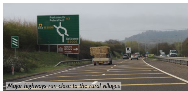
Ineffective and intrusive traffic engineering - Blackmoor
