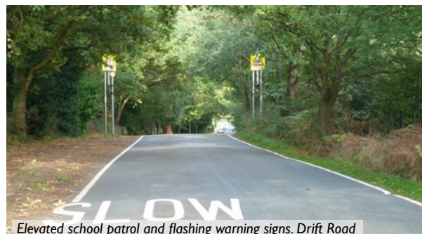
Elevated school patrol and flashing warning signs. Drift Road
