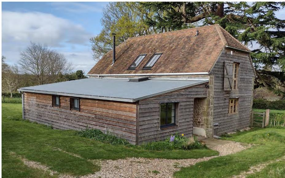
Sympathetic conversion of a traditional stone Sussex Barn into a 3 bedroom dwelling. The Barn was built in 1810 from local stone with a clay plain tile roof and had a lean-to open sided cart shed side extension; it remained largely unaltered until its last use as a lambing shed for the former St Cuthman's School until it closed.
