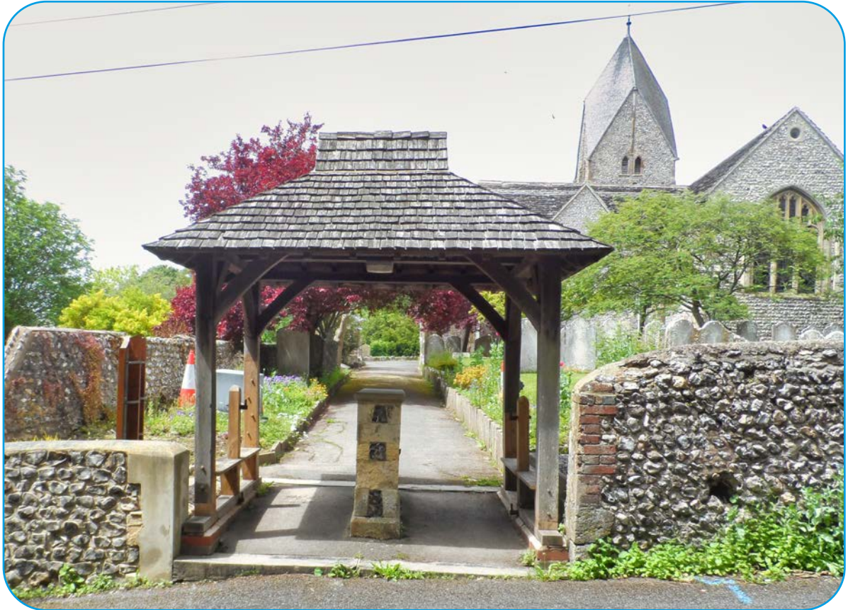
A typical lychgate stands at the entrance to the churchyard. Prior to the start of a funeral, coffins were often kept under the lych gate and, as here, a central pier was provided on which to rest the coffin.
