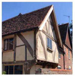
Rotted frame sections have been sensitively replaced by splicing new sections, with an emphasis on retaining as much of the original fabric as possible. Wattle and daub panels, some thought to be original, have also been repaired. Those panels that had failed were re-panelled using a remix of the original daub. A period window has also been added to the original, second storey 'solar', after evidence was found in the timber-frame of a previous window aperture in that location.
