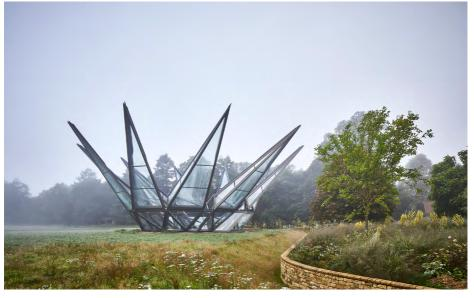
A feature kinetic glasshouse, 15 metres high, at Woolbeding National Trust Gardens made up of ten openable segments (sepals) designed to open and close in the manner of the opening and closing of a flower. The glasshouse is the focal point of expansion of the formal visitor gardens at Woolbeding, with the creation of a natural pathway and planting narrative charting a route through the 'Flora of the Silk Road'.
