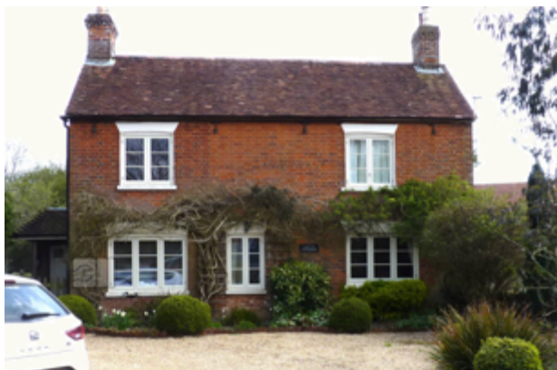
Photo 29. Laurel Cottage in plain red brick
