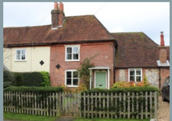
Photo 33. Cottages in Queen Street displaying walls of painted brick, plain red brick (unpainted) and flint and brick.
