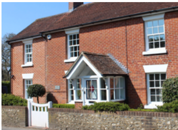
Photo 34. Sash windows with deep stone cill and frames set behind brickwork at Yew Tree Cottage
