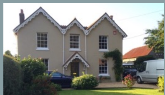
Photo 28. Gable ends facing the road are unusual in the village. The decorative barge boards are also not typical but add to the visual variety in the street.
