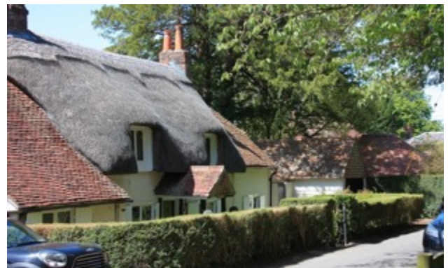
Photo 23. Little Croft on Church Street showing a variety of traditional building materials including thatch, clay plain roof and wall tiles, painted brick, and timber boarding.
