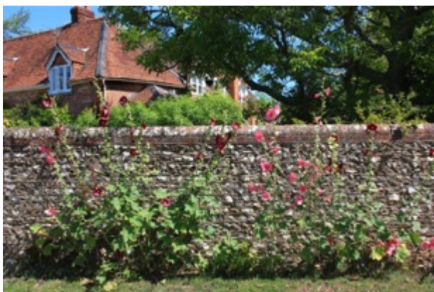
Photo 15. Flint and brick boundary wall in Shoe Lane.
