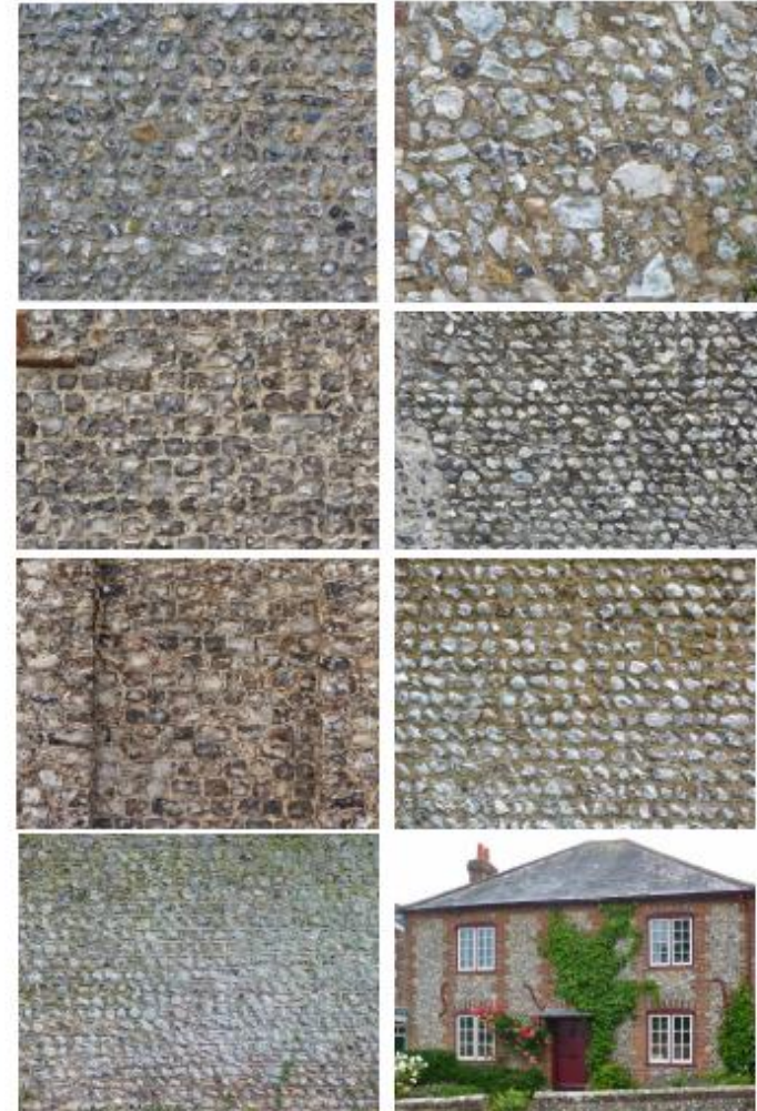
Figure 14: The appearance of the flintwork varies throughout the village; the panels above show some of this variety, which ranges from fairly rustic through to quite fine and includes some examples of galleting. The irregular nature of most flint requires the use of an alternative material to form corners. In Slindon this is almost invariably brick and it is often used in a distinctive fashion in which the brickwork jambs of the ground floor and first floor windows/ doors are continuous.
