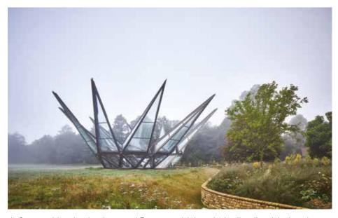
A feature kinetic glasshouse, I5 metres high, at Woolbeding National Trust Gardens made up of ten openable segments (sepals) designed to open and close in the manner of the opening and closing of a flower. The glasshouse is the focal point of expansion of the formal visitor gardens at Woolbeding, with the creation of a natural pathway and planting narrative charting a route through the 'Flora of the Silk Road'.
