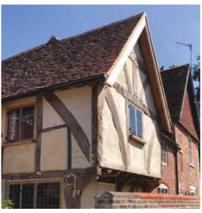
Rotted frame sections have been sensitively replaced by splicing new sections, with an emphasis on retaining as much of the original fabric as possible. Wattle and daub panels, some thought to be original, have also been repaired. Those panels that had failed were re-panelled using a remix of the original daub. A period window has also been added to the original, second storey 'solar', after evidence was found in the timber-frame of a previous window aperture in that location.
