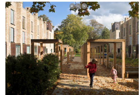
Figures 10, 11 and 12: Top: Garage and vehicle workshop in Andelfingen - Lüchinger + Meyer Bauingenieure AG. Middle: Workshop Building in Mechelen - dmva. Bottom: Accordia, Cambridge - Mole Architects
