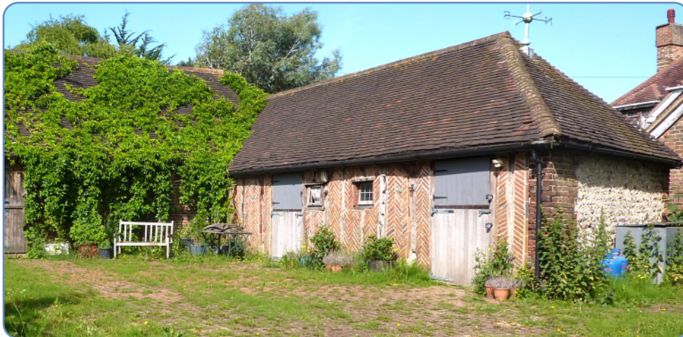
Former Stables of Dyke Farm, worthy of local heritage recognition
