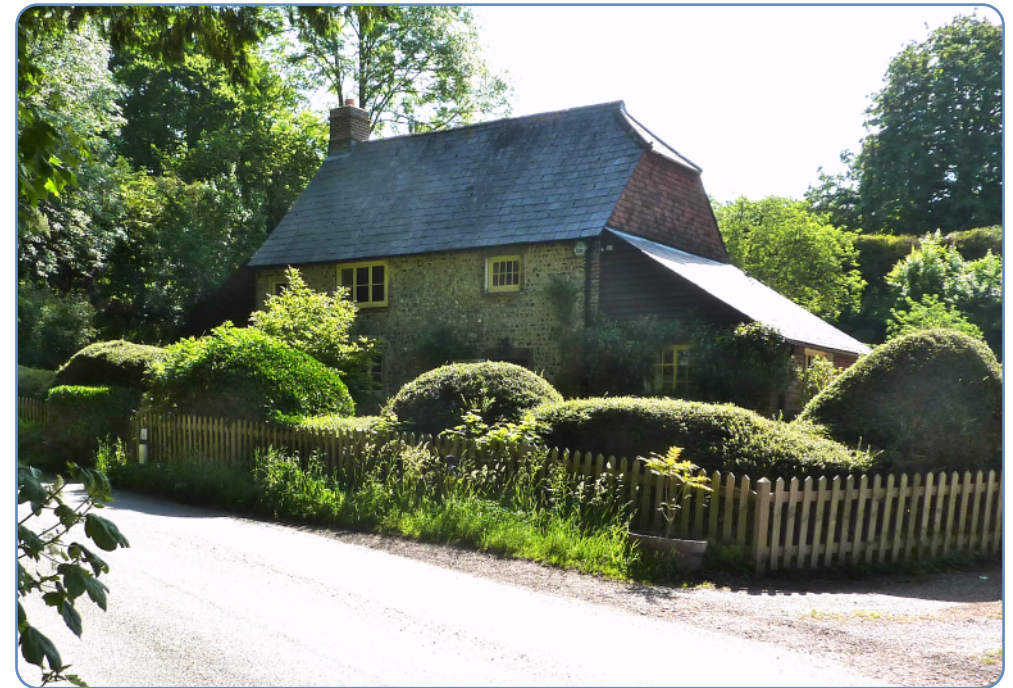
Glebe Cottage (above) is a vernacular cottage of the Seventeenth Century faced in flint and listed at Grade II
