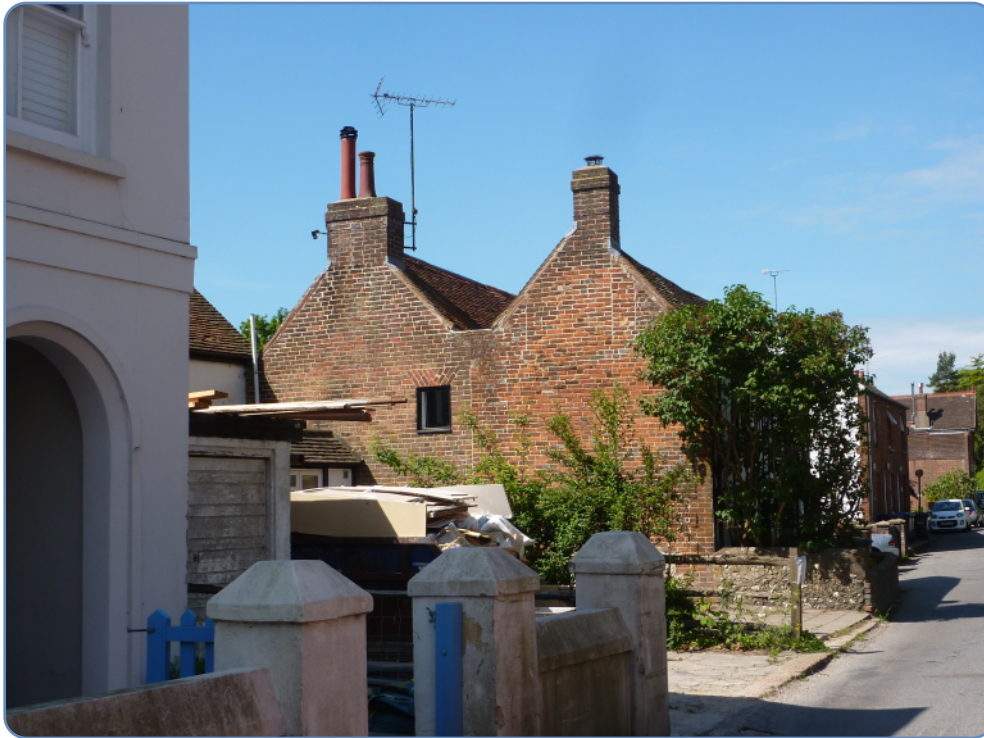
The south side of The Street has a slightly disjointed appearance due to a markedly varied building line. Some cottages, originally set back for cottage gardens, now provide parking spaces or garaging, to the detriment of the street scene.
