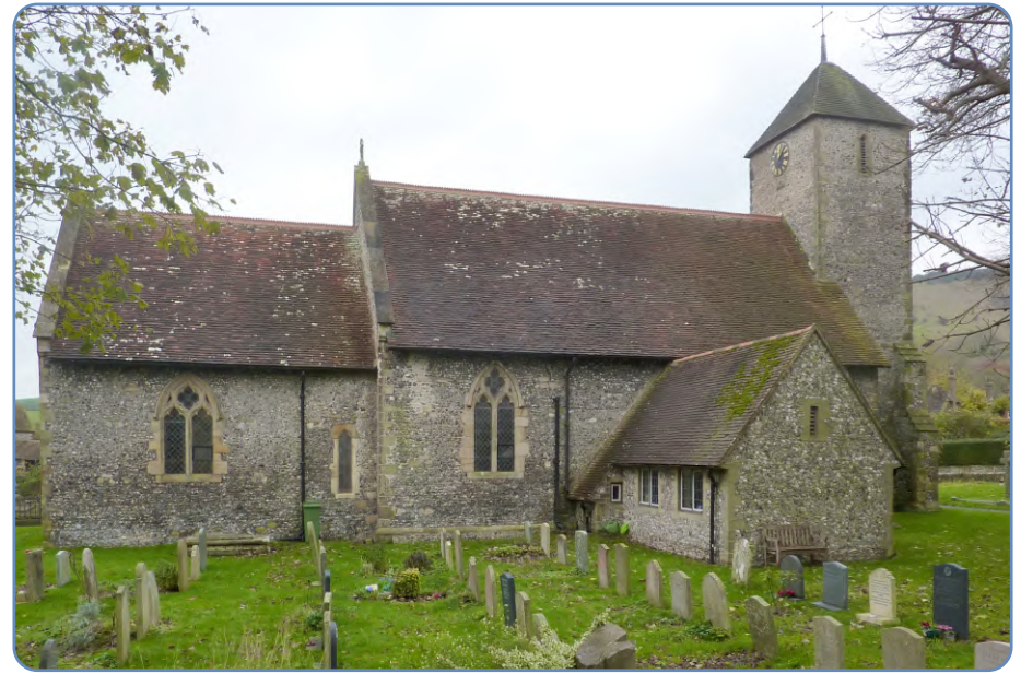
Figure 17: The Parish Church of St Pancras.
