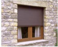
Security shutters are installed on the outside of windows and offer a more robust method of preventing light spill.
