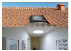
If illuminating indoor spaces solely with sunlight is required, then light tunnels – effectively oversize fibre optic cable – can be alternative to larger skylights.
