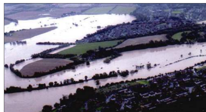
PHOTOGRAPH OF THE NORTH END OF THE APPLICATION SITE DURING FLOODS IN 2000
