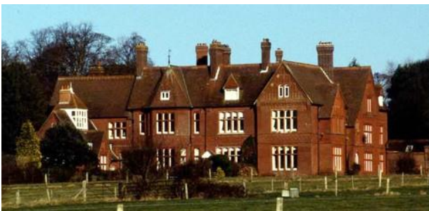
Above: Swanmore Park House, designed by Alfred Waterhouse and now divided into separate dwellings.
