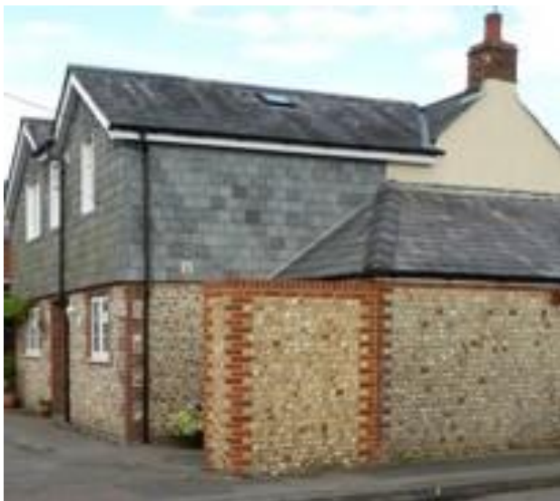
Below: Sympathetic extension to a traditional flint wall in the heart of the village.
