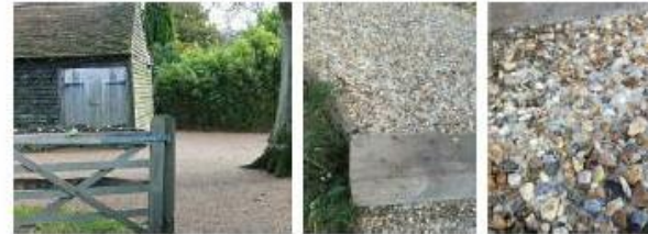
Examples of porous mortar bound gravel, made on site.
