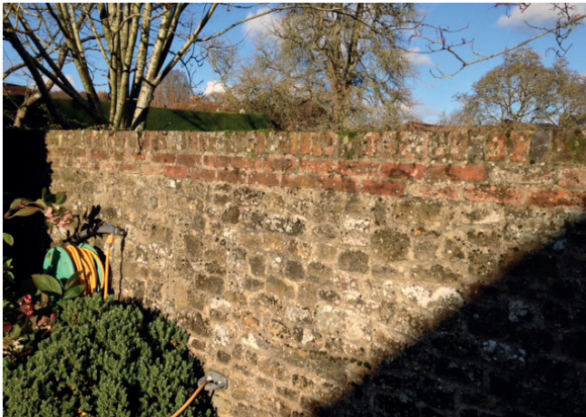
Typical local stone and brick wall in residential car park (Midhurst)
