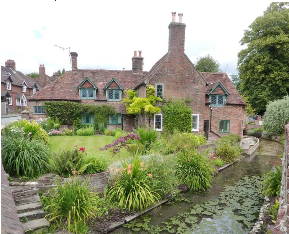
Figure 58: Mill House , Warnford Road. Mill and House. 18 th century in date with late 19 th century extensions and alterations.
