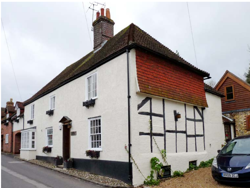
Figure 38: The Baechus , East Meon Road. An early 19 th century brick facade hides a 17 th century or earlier timber frame which is still exposed on the gable end.
