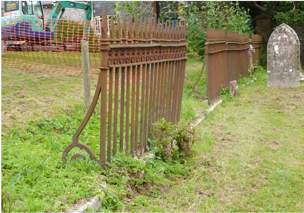
Figure 22: Railings and gates in the churchyard.
