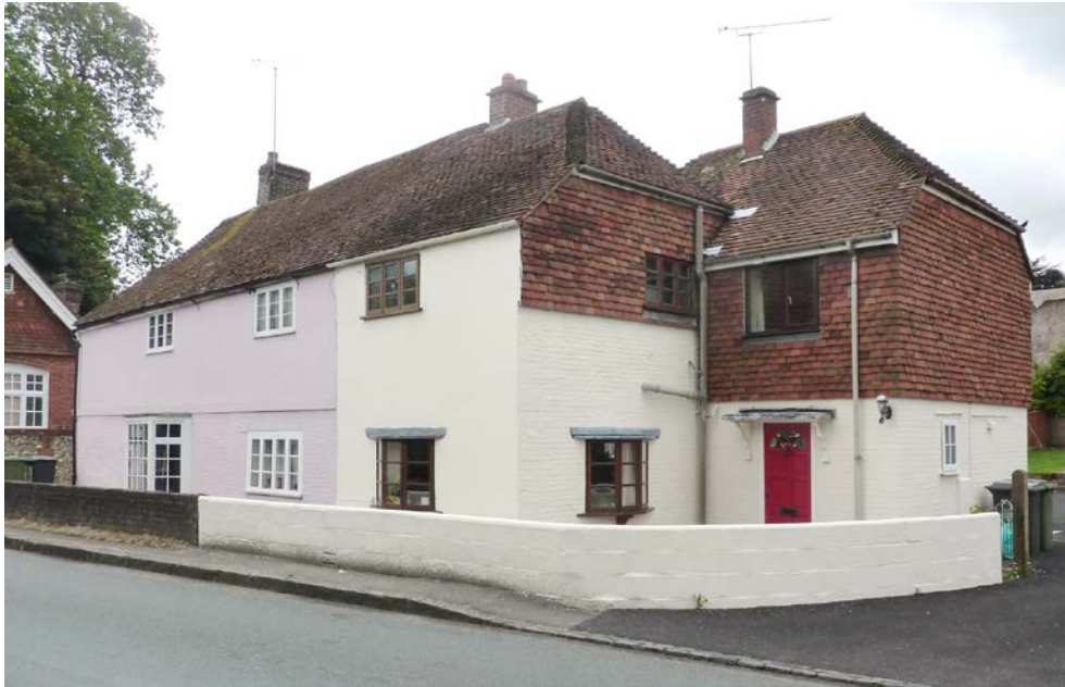
Figure 16: Rose Cottages , Warnford Road, of timber-framed origin but re-clad in the early 19 th Century.
