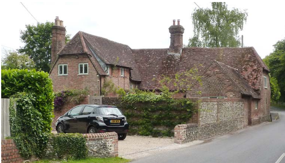
Figure 49: Shafts House , East Meon Road. Timber-framed in origin and clad in brickwork in the 18 th century
