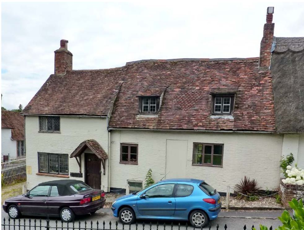
Figure 30: The Cross Cottage , Church Lane
