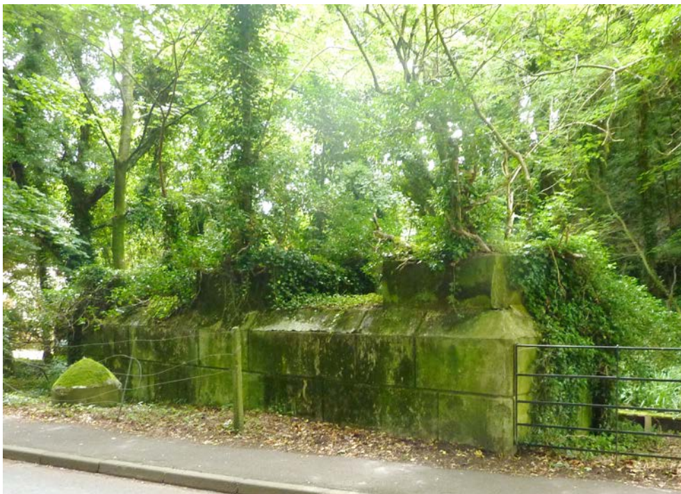
Figure 47: One of the surviving concrete piers from the former railway viaduct. The iron superstructure would have dominated the valley between 1903 and its removal in the 1960s, following closure of the line.
