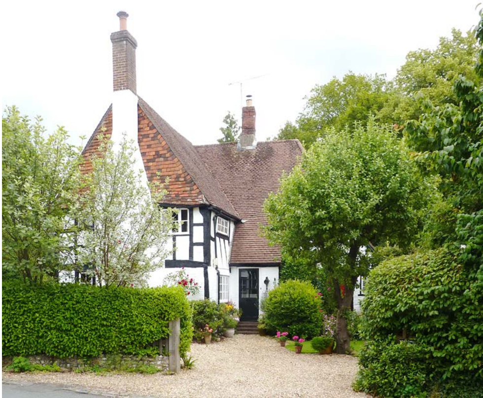
Figure 57: Hatch Cottage , Warnford Road. The 17 th century timber frame remains visible on the front but the back was clad in the early 19 th century.
