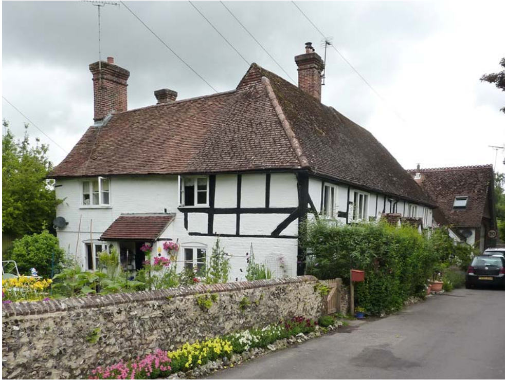
Figure 14: 1, 2 and 3 Station Road. Originally a single dwelling of late 16 th century origin, with 19 th Century rear extensions. The steeply pitched main range was originally thatched.
