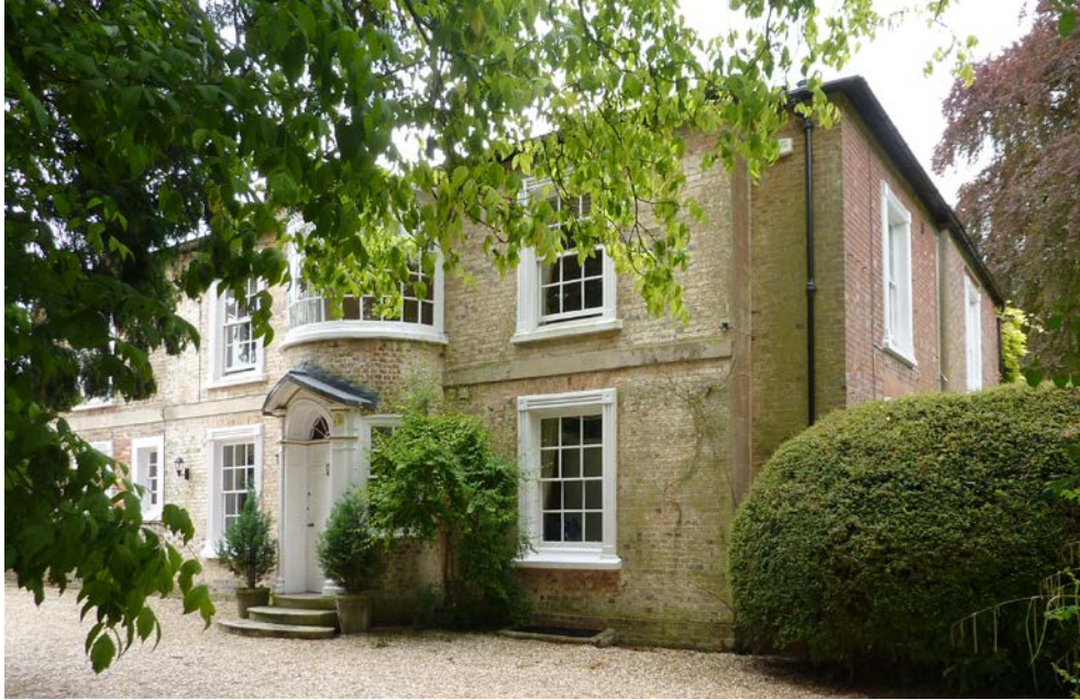
Figure 18: West Lodge , Warnford Road. House and service wings of early, mid and late 19 th century date. The semi-circular two-storeyed central bow on the front elevation, incorporating a classical doorcase, is a particularly attractive and unusual feature.
