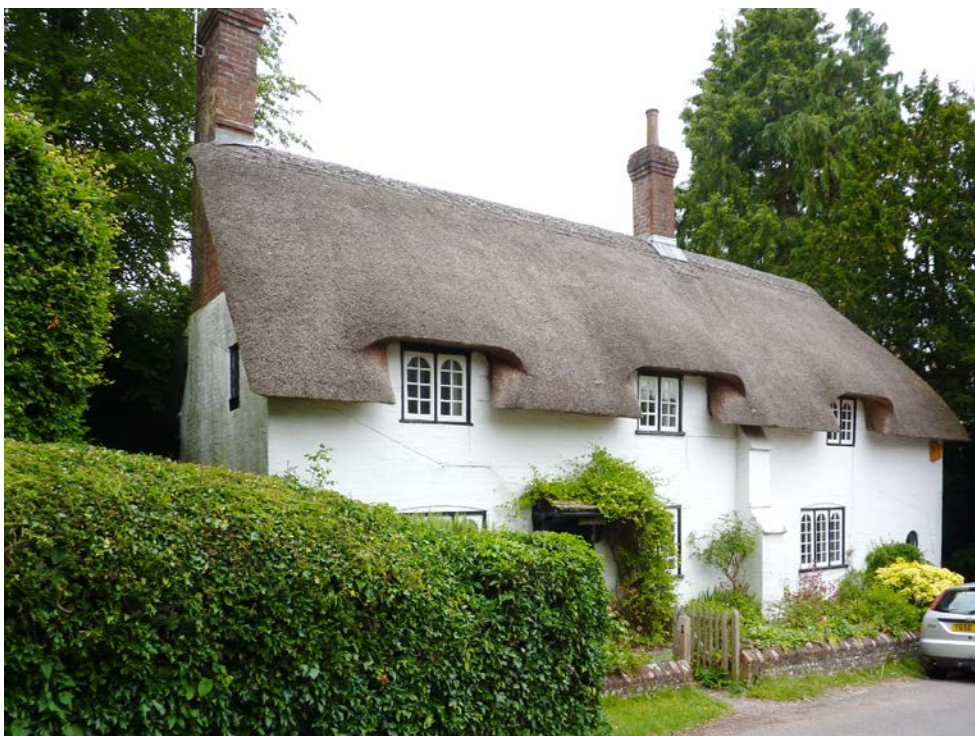
Figure 26: Culverkeys , Church Lane. A late 18 th century cottage.
