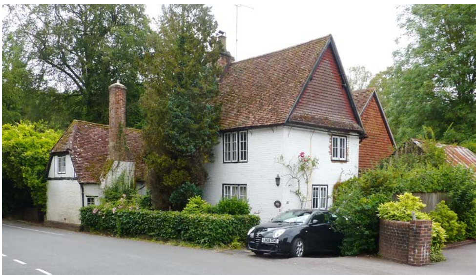
Figure 36: Brook Lodge and Gobions , East Meon Road. A 17 th century timber framed core with late 18 th , early 19 th and 20 th century extensions
