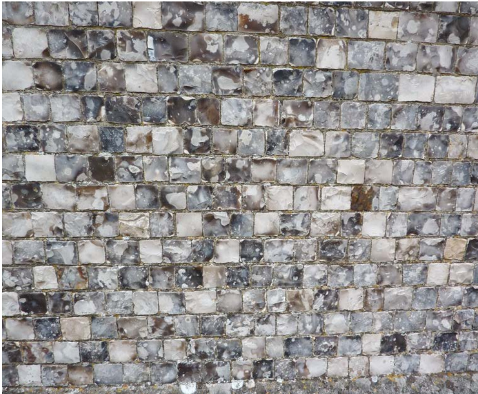
Figure 21: very high quality flintwork, using squared and coursed, knapped flints.
