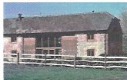
Barn conversion, Church Lane.
