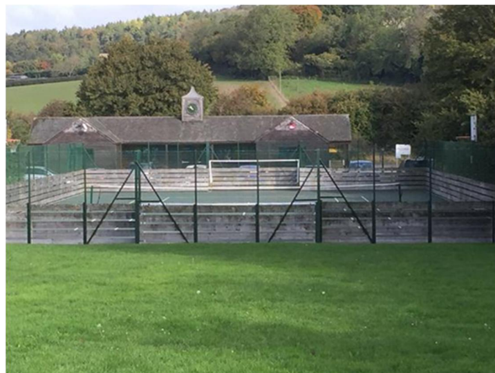
Multi-Purpose Sports Court & Sports Pavilion
