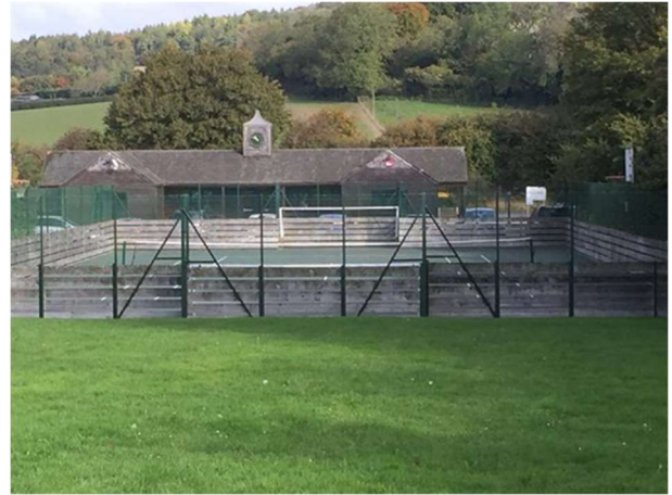
Multi-Purpose Sports Court & Sports Pavilion
