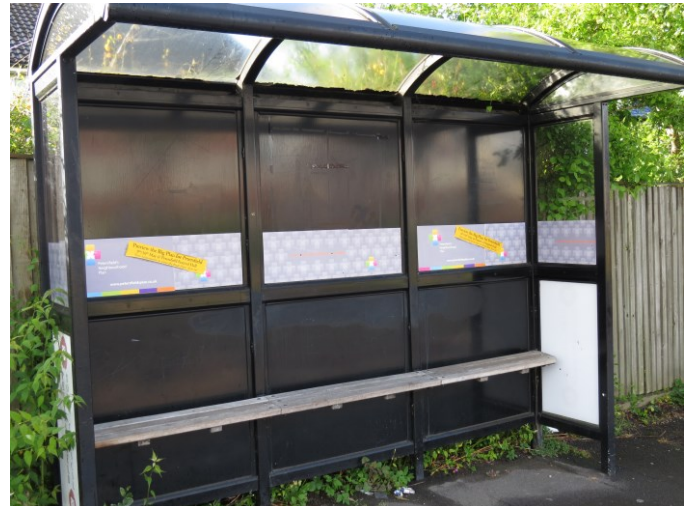
Figure 7 - Bus Stop Shelter PNP Branding
