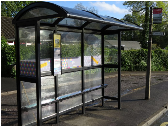
Figure 6 - Bus Stop Shelter PNP Branding
