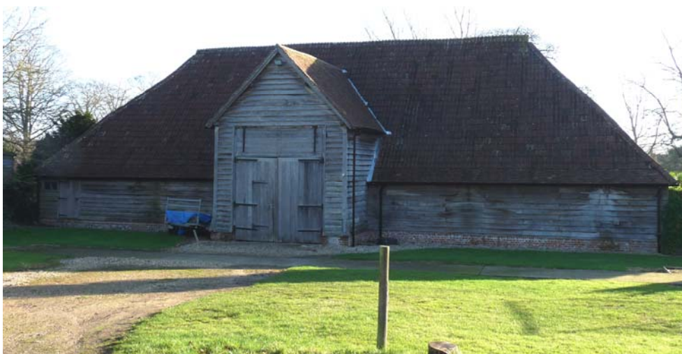
Figure 25: Barn 60 metres north-east of Exton Farmhouse
