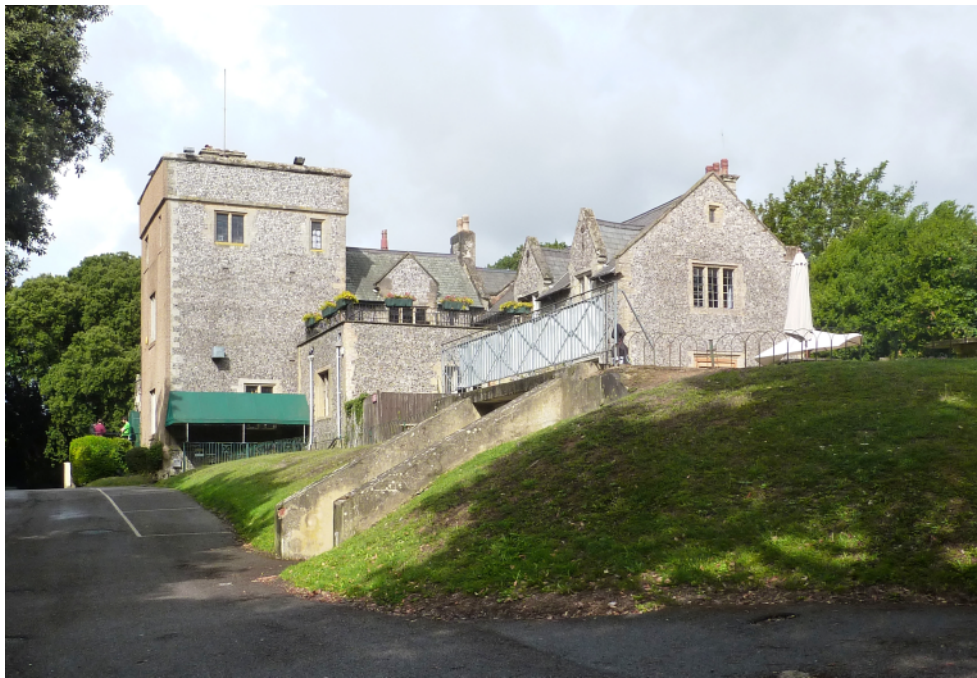
Figure 7: Highdown Tower from the south-east before (above) and below (after) the recent works. The removal of the green canopy and the painting of the railings have both improved the appearance and setting of the hotel
