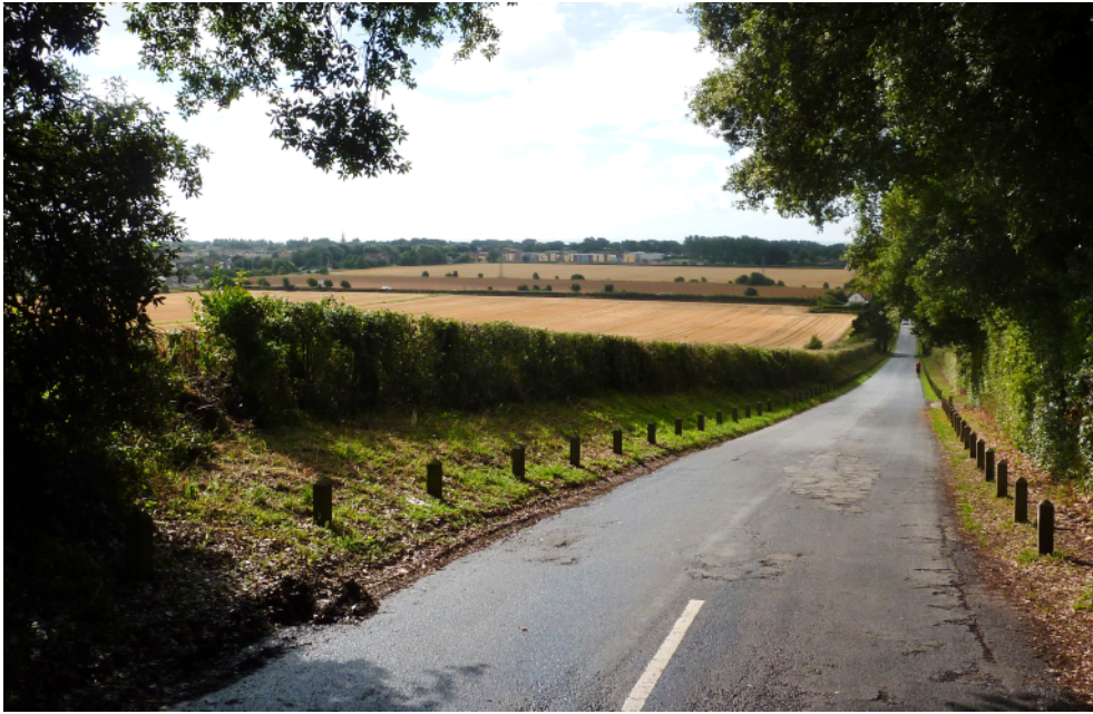
Figure 6: Views out from the Conservation Area to the surrounding landscape are few but the main exceptions is this view from the top of the drive. The poor condition of the road surface can be seen in the 'before' shot above and the improved surface in the 'after' photograph below.
