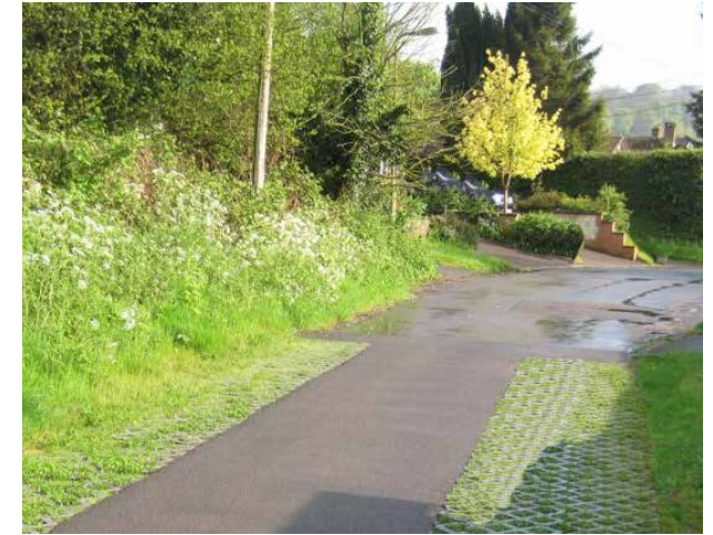
Reinforced grass paving forms soft verge - Buriton
