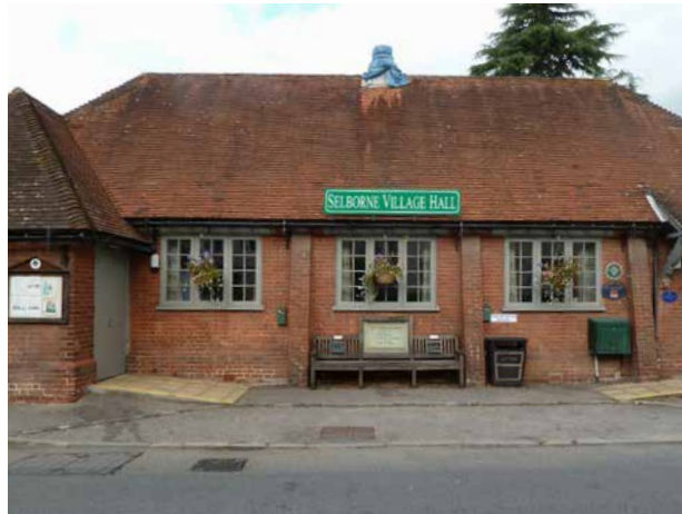
The village hall opposite local shops could combine with highway design to slow traffic through place-making
