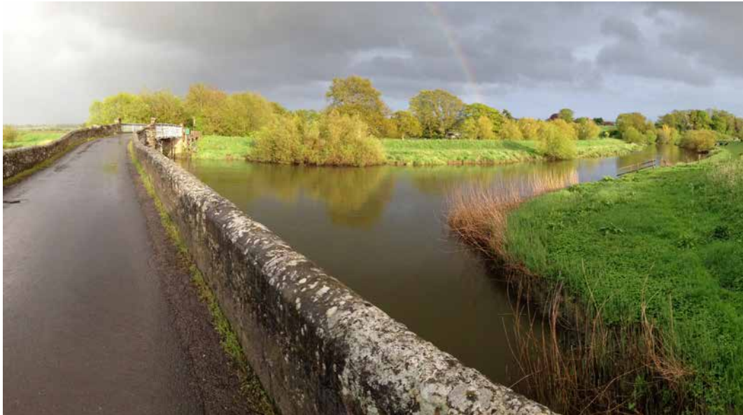
The National Park's roads and bridges form an integral part of its landscape. Greatham Bridge, Pulborough
