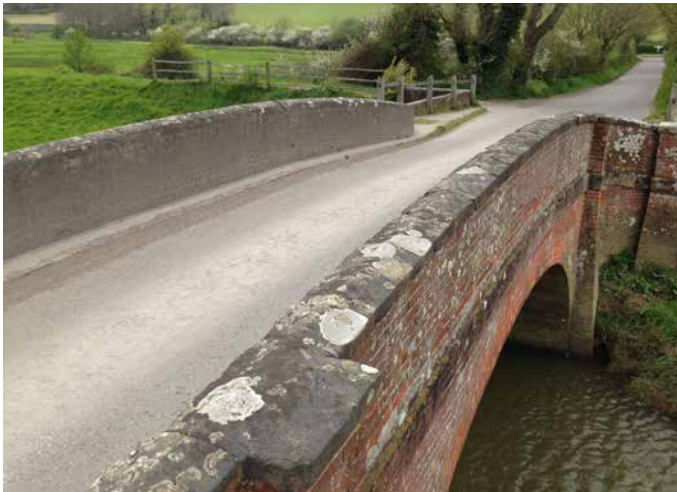
A simple elegant arched bridge punctuates a road
