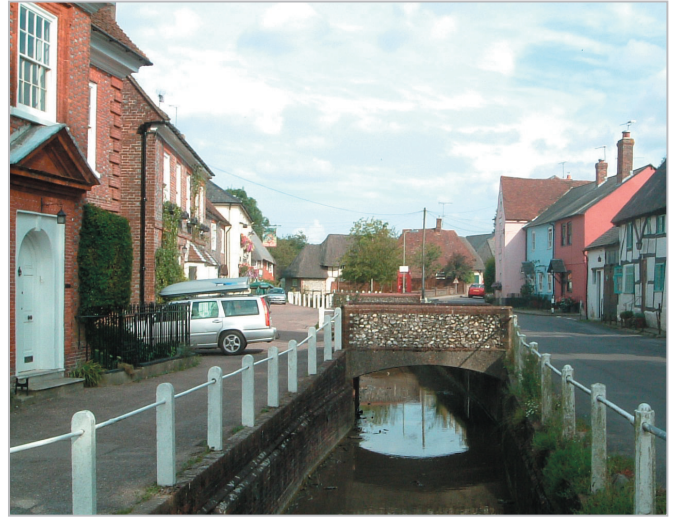
Frequent river crossing points on historic bridges.
