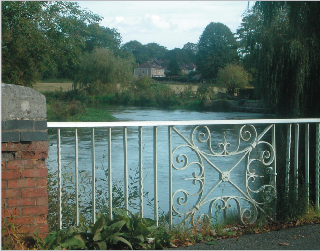
Frequent minor river crossing points are marked by white bridges.
